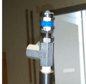
Figure 4.5. Pressure relief valve
