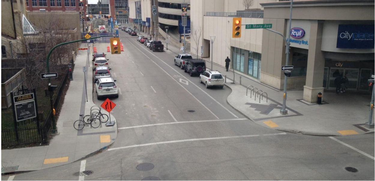
Figure 7: Existing Curb Extension at Hargrave and St. Mary (November, 2016)
