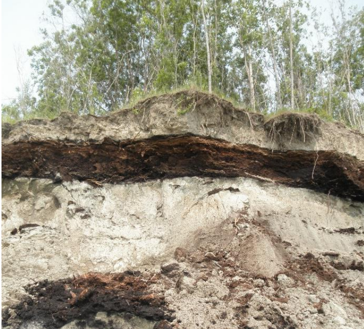
Figure 3.2 Photograph of the 2-Mile Channel outlet, displaying slumping and signs of subsurface soil contamination from falling organic material, August 2014.
