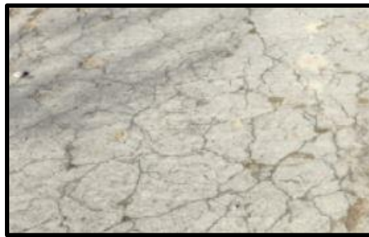
Figure 2.5: Map crazing/ cracking
