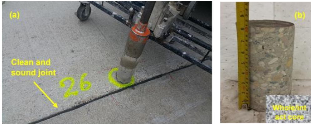
Figure 4.3: An example from a residential street showing: (a) sound joint without evidence of faulting or spalling, and (b) whole/intact core.
