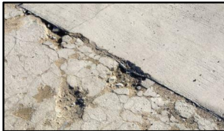
Figure 2.4: Joint Spalling
