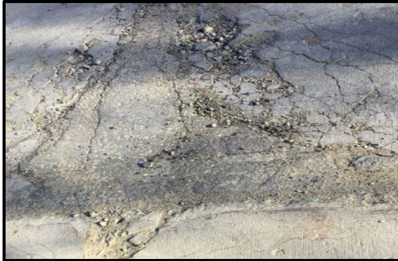
Figure 2.1: D-cracking of concrete pavement.
