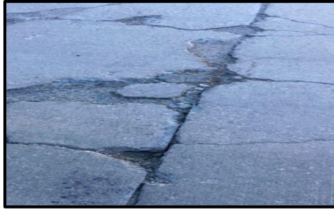
Figure 2.7: Joint deterioration of concrete pavement
