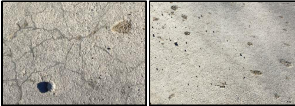
Figure 2.3: Pop-out at concrete surface.
