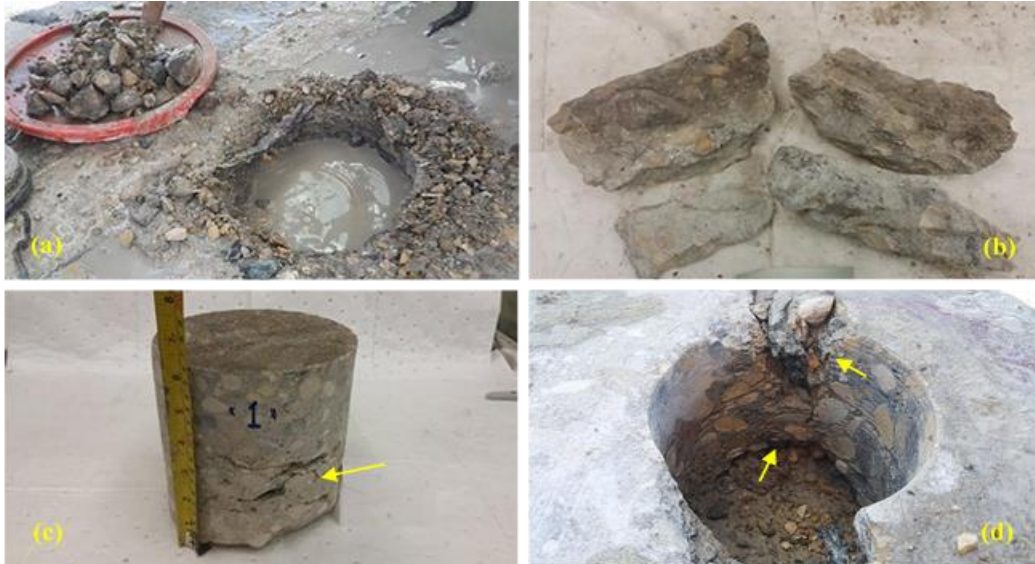
Figure 4.2: An example from regional roads showing: (a) damage of concrete during the coring process, (b) fractured cores, (c) sub-parallel cracks in the extracted cores, and (d) damage of top and bottom parts.
