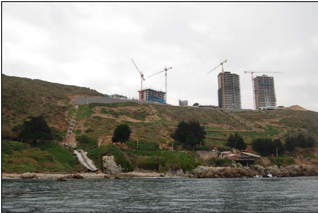
Figure 4.3: Real estate developments and the storm sewer outlet (on the left) discharging over Montemar's MA.
