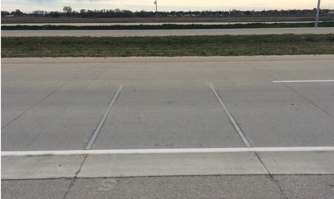
Figure 6: Piezo-quartz sensors installed at WIM Station 99 on Manitoba's PTH 190. Photo taken by Steven Wood on October 9, 2016.
