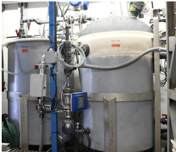
Figure 8 ANITA™ Mox Pilot, showing BOD removal reactor (left), deammonification reactor, piping, valves, mixer and heater (Wilson, et al. 2015)
