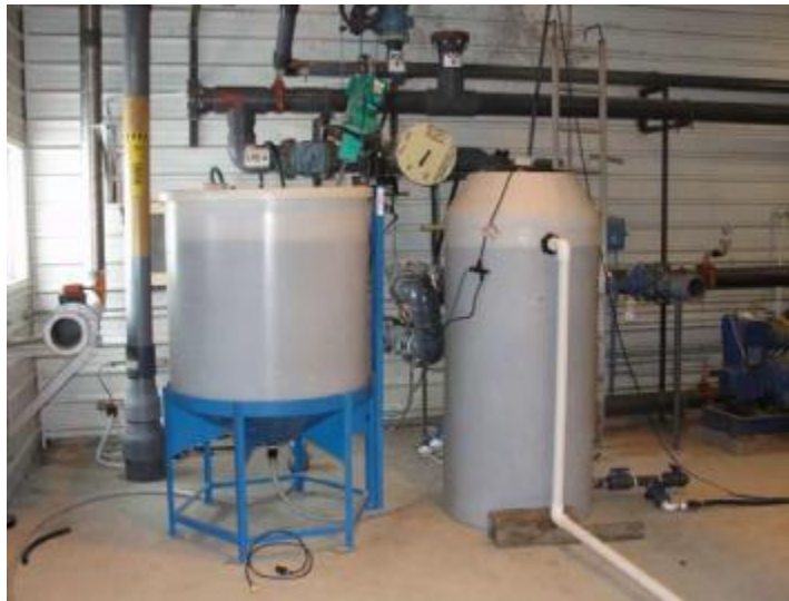
Figure 7 Equalization and Blending Tanks
