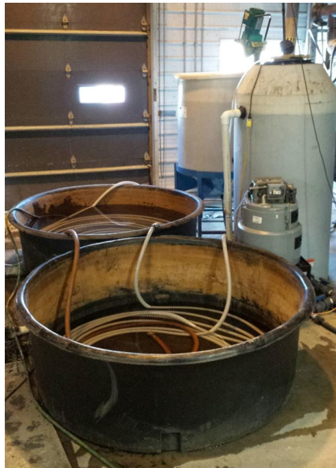
Figure 9 Heat exchanger for low temperature phase
