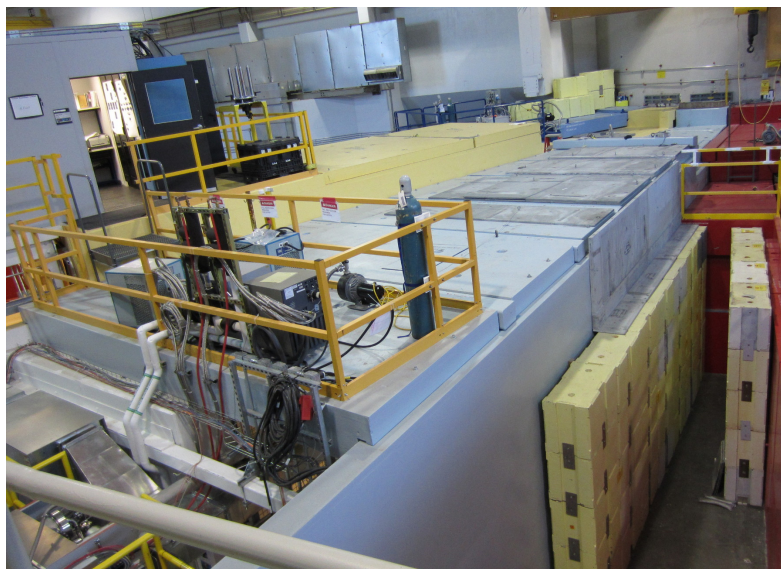
Figure 2.5: The exterior of the FnPB cave. Only the concrete shielding is visible. The FnPB beamline shielding is painted light blue while the adjacent beamlines are yellow and red.
