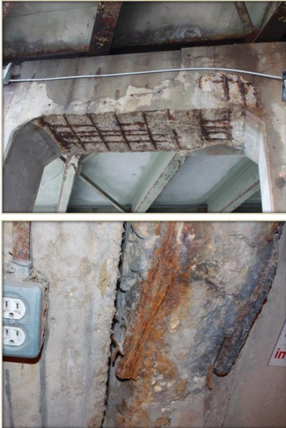
Figure 2.3: Corrosion in a bridge structure.
