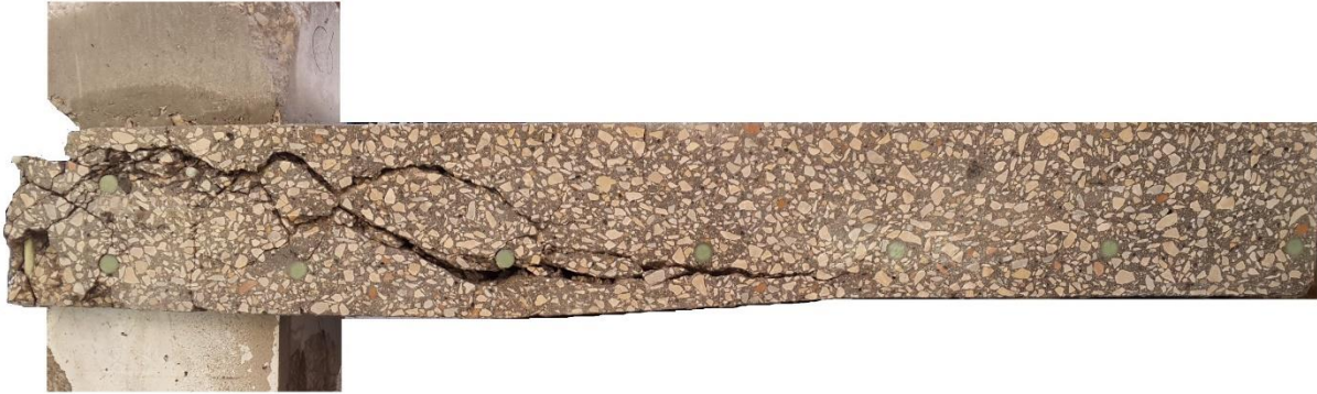
(a) Internal cracks for connection N-0.9-C6
