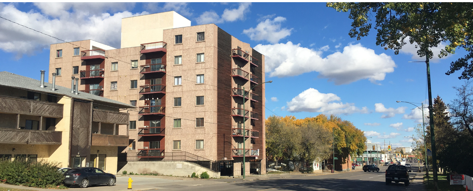
FIGURE 17: Site Context North East
