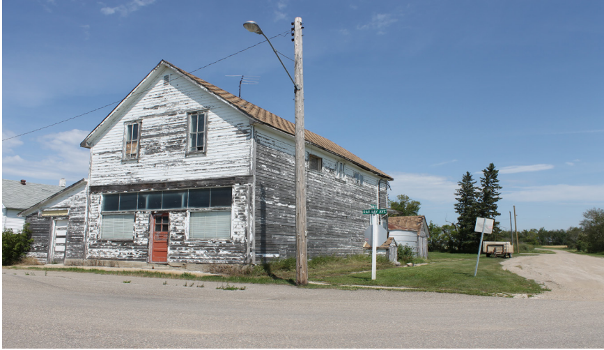
1 Main street building in disrepair.
