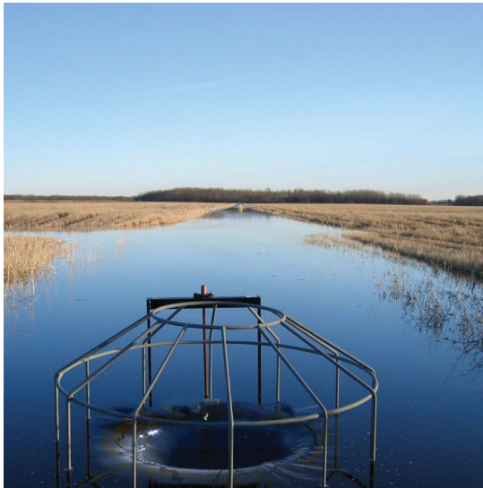
1.2 The Waffle® concept water intake site with protective cage. (Image: Kurz et al., 2008)
