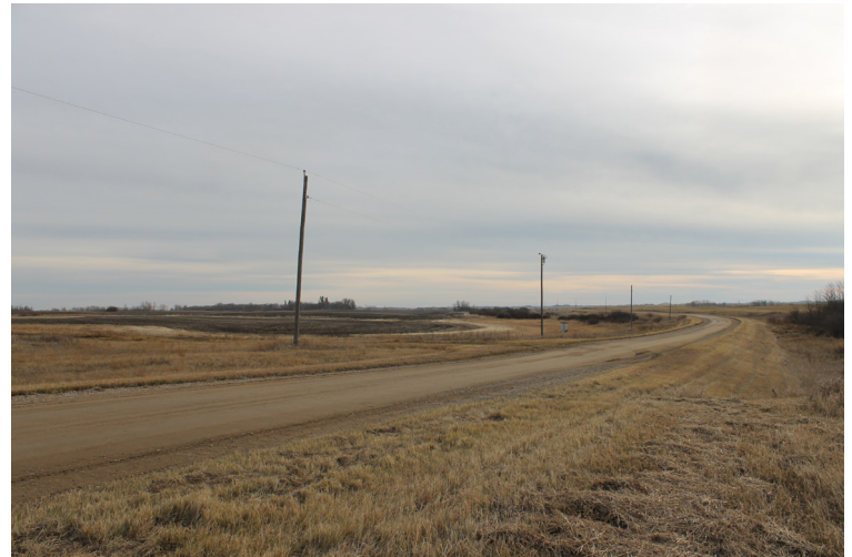
4 Elevated roadway south of Cardale.
