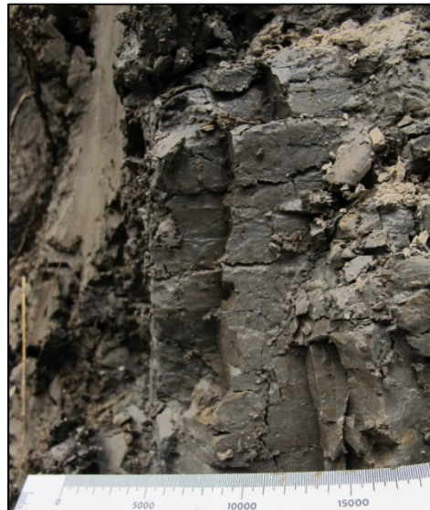
Figure 3-14. Fissured clay foundation from Test Pit 2 at depth = 7 ft.
