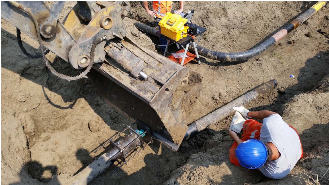
Figure 4-22 Excavator Pushing on Abandoned Pipe.
