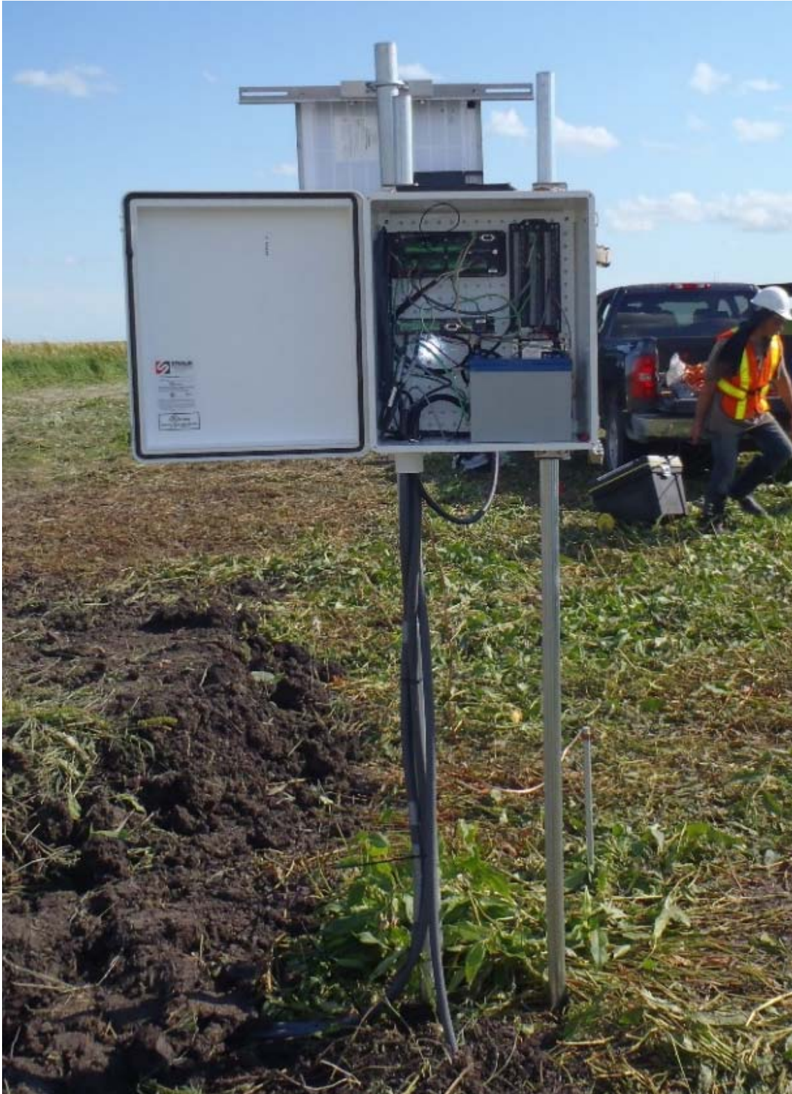
Figure 4-18 Data Acquisition (DA) System, with auxiliary components and Solar Panel Set-Up.
