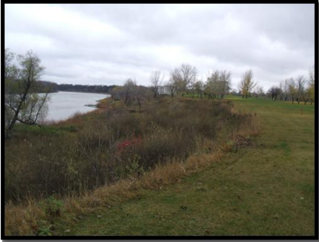
Figure 3.10: Typical failure controlled bank along the Red River on an outside bend. Note the retrogressing headscarp and shallow slope angle.
