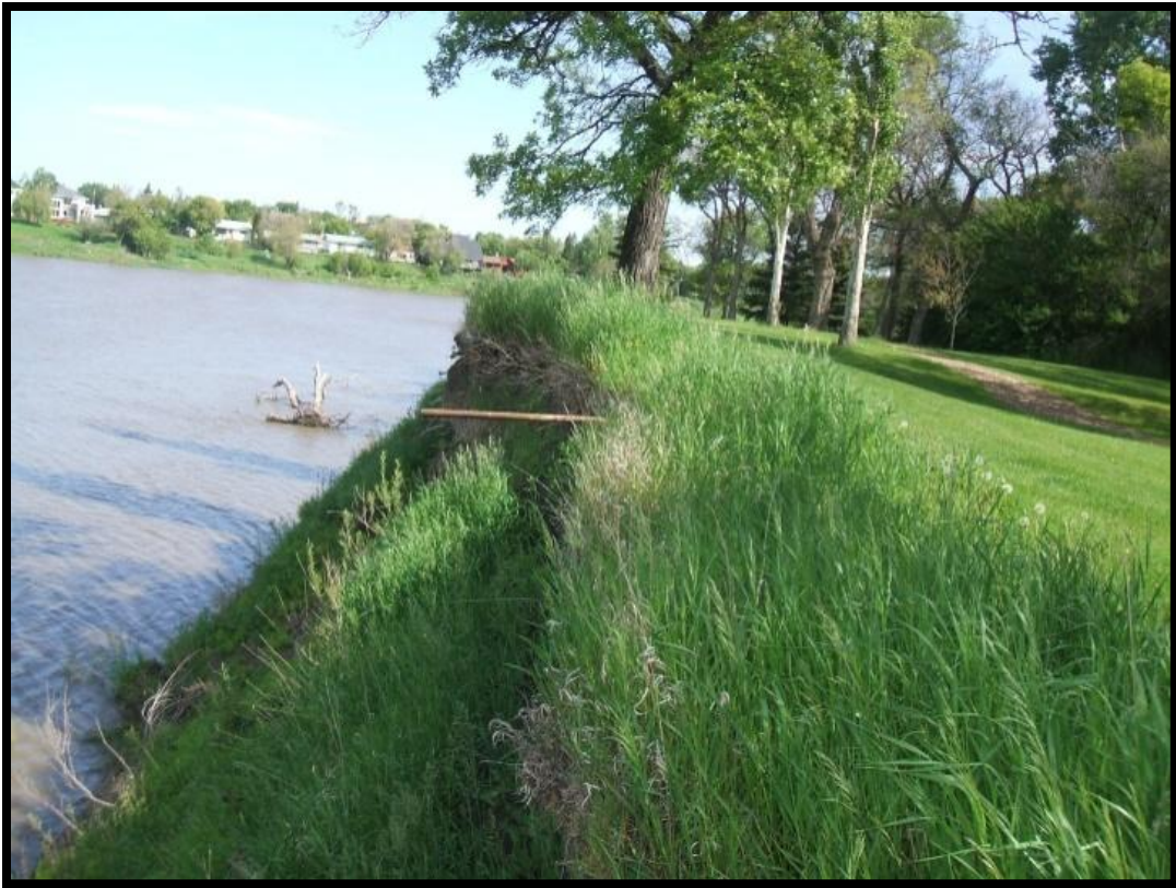
Figure 3.11: Typical erosion controlled bank encountered along the inside bend of the Red River. Note the steep riverbank face.
