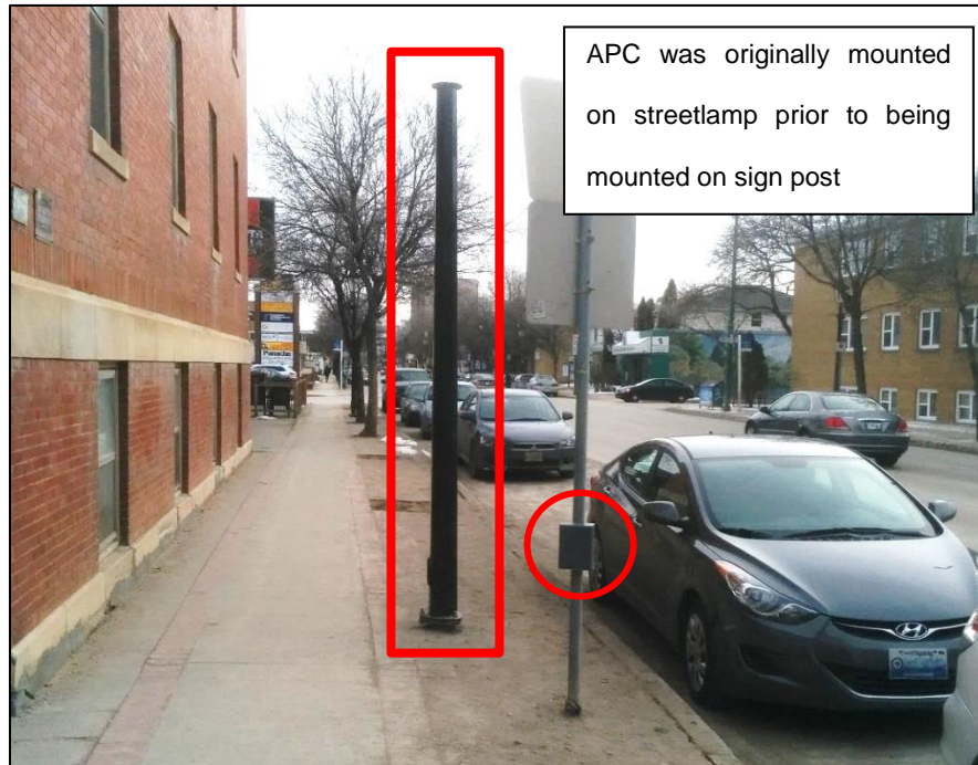
Figure 11: Streetlamp (and APC) Removed by City during Maintenance
