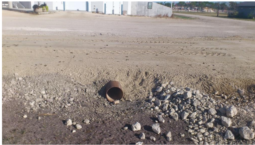
Figure 3.1 Preparation of storage site for silo bag storage system
