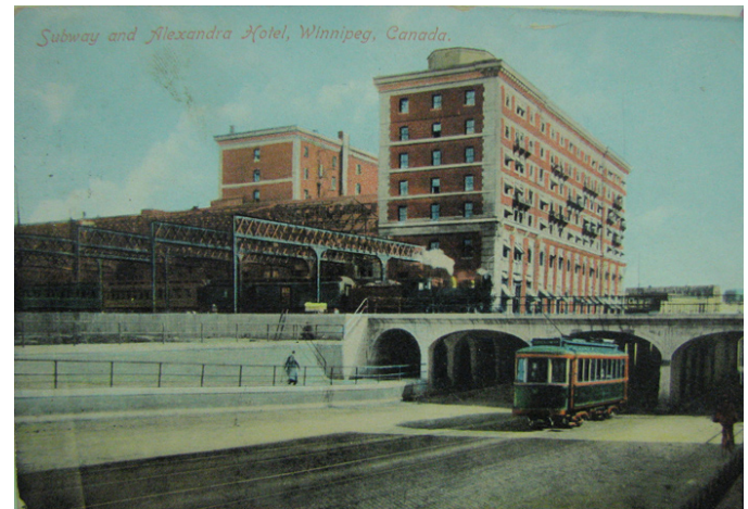
Figure 8.03 -The underpass at Main Street was a major improvement over the on-grade railway crossings. In the background, the Royal Alexandra Hotel greeted visitors as they arrived in the bustling city centre.
