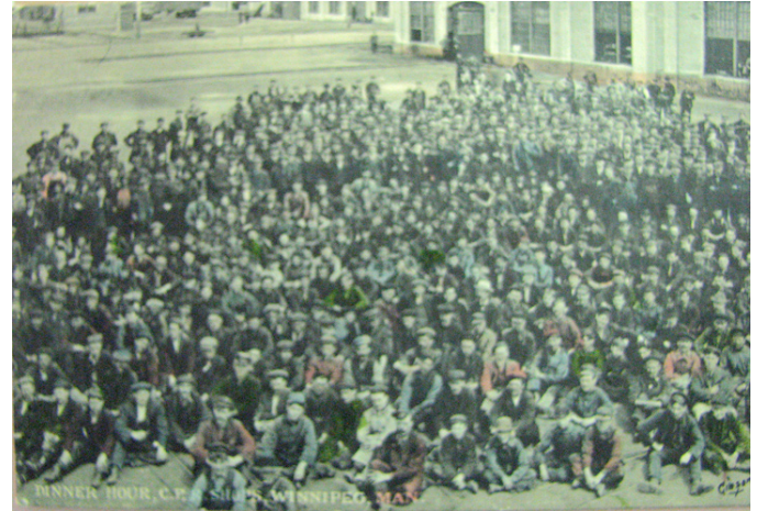
Figure 8.04 - An early photograph of Winnipeg CPR workers, many of whom were new immigrants to the city. Many of these men would have purchased or rented homes in the North End where the CPR built and owned worker housing.
