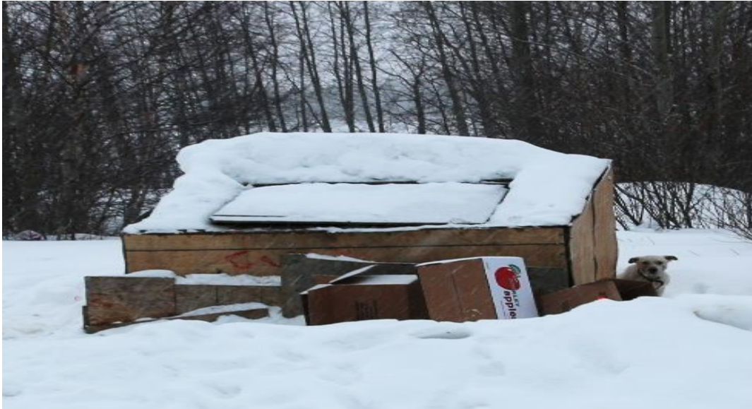
Figure 4.11: A stray dog wandering around a wooden waste container: wooden bins are easy to construct locally but are fragile and easily destroyed by weather and animals in search of food.
