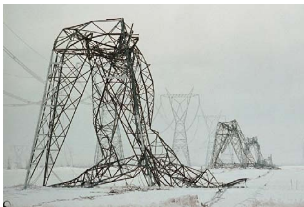
Figure 11: Hydro pylons bend and break from weight of ice during Montreal ice storm (IceStorm, Robert Lebarge photographer, 2005. Used with permission.)
