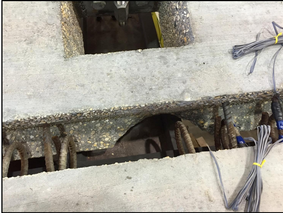
Figure 3-22 – Damage to Bottom Lip of Joint (East Joint of TS2 – Panel E2) During Placement
