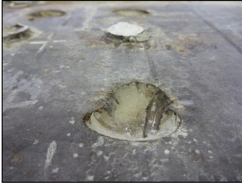
Figure 4-23 – Close-up of Damaged Shear Stud Weld (Test #2)
