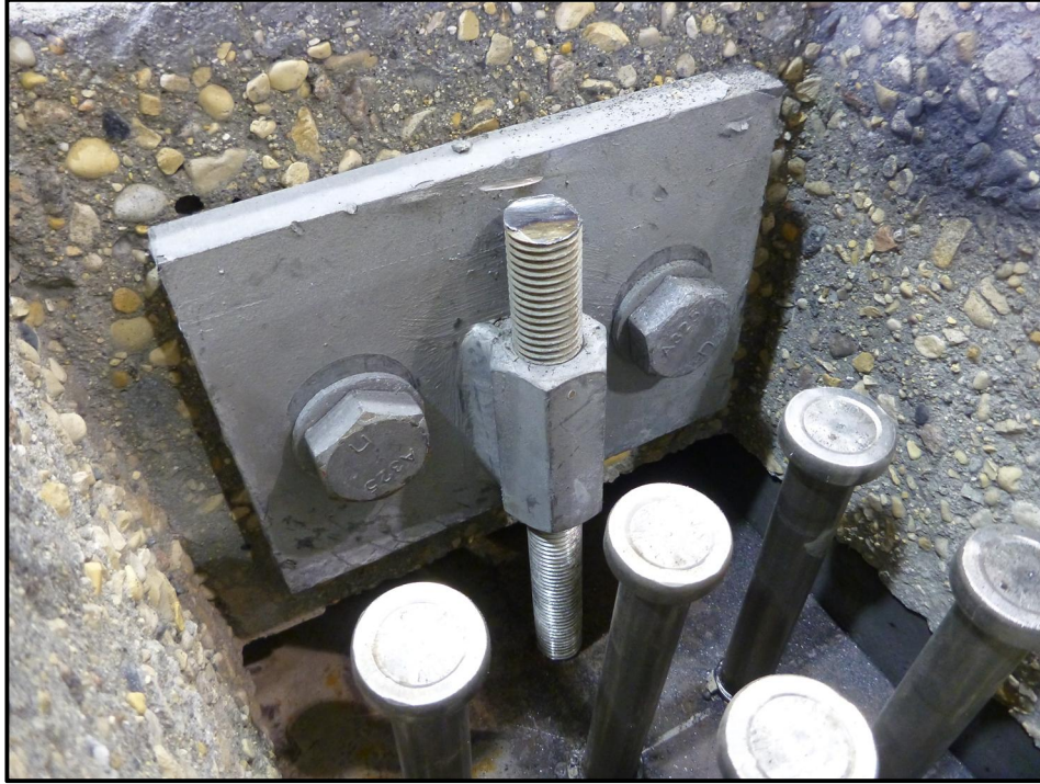
Figure 3-14 – Typical Leveling Plate and Bolt (Head of Bolt Cut Off Prior to UHPC Casting)
