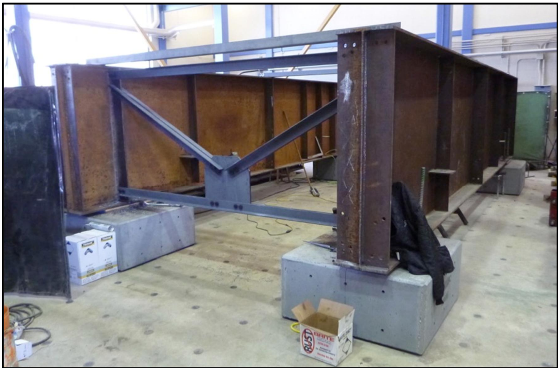
Figure 3-4 – Steel Plate Girders and End-Diaphragm Installation (TS1) [Typical]
