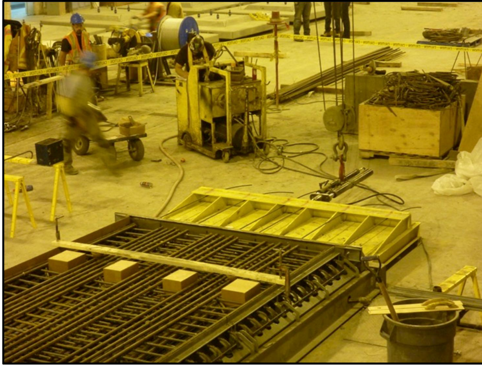
Figure 3-10 – Stressing of Strands
