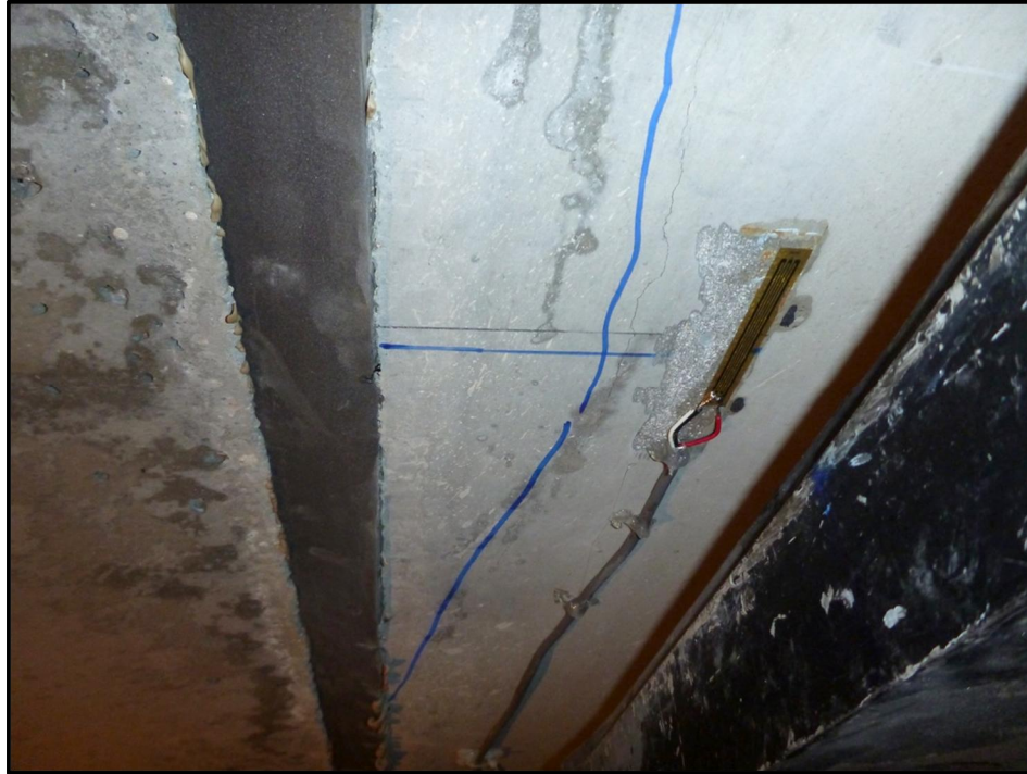
Figure 3-37 – ESG Installed on Concrete Prior to Protective Coating
