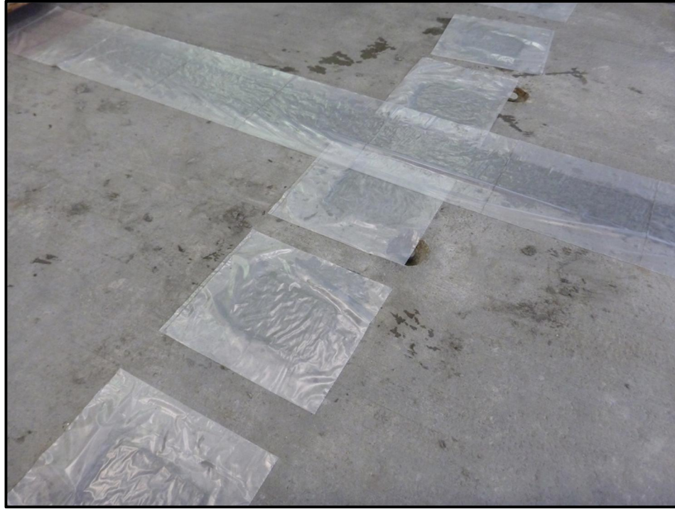
Figure 3-27 – UHPC Joint and Shear Pockets Covered with Poly
