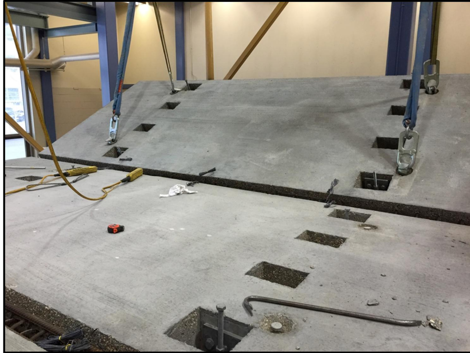
Figure 3-20 – Placement of TS2 Panels Utilizing Steep Tilt
