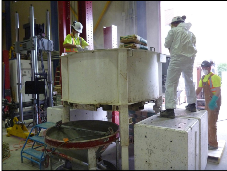
Figure 3-25 – Mixing of UHPC
