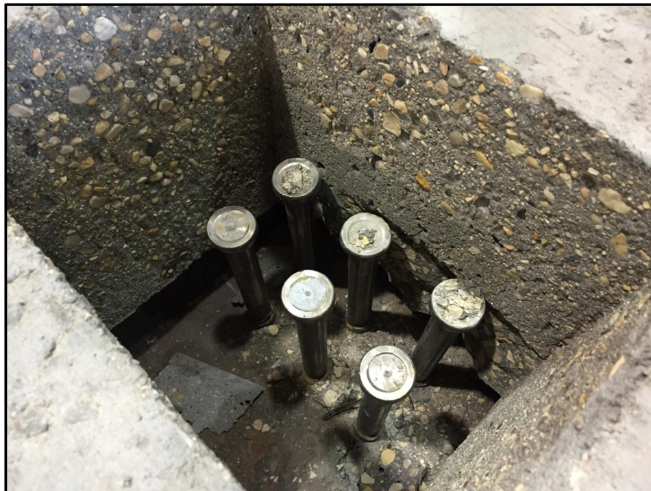
Figure 3-21 – Damage to Inside Face of TS2 Shear Pockets (Panel C2) During Placement
