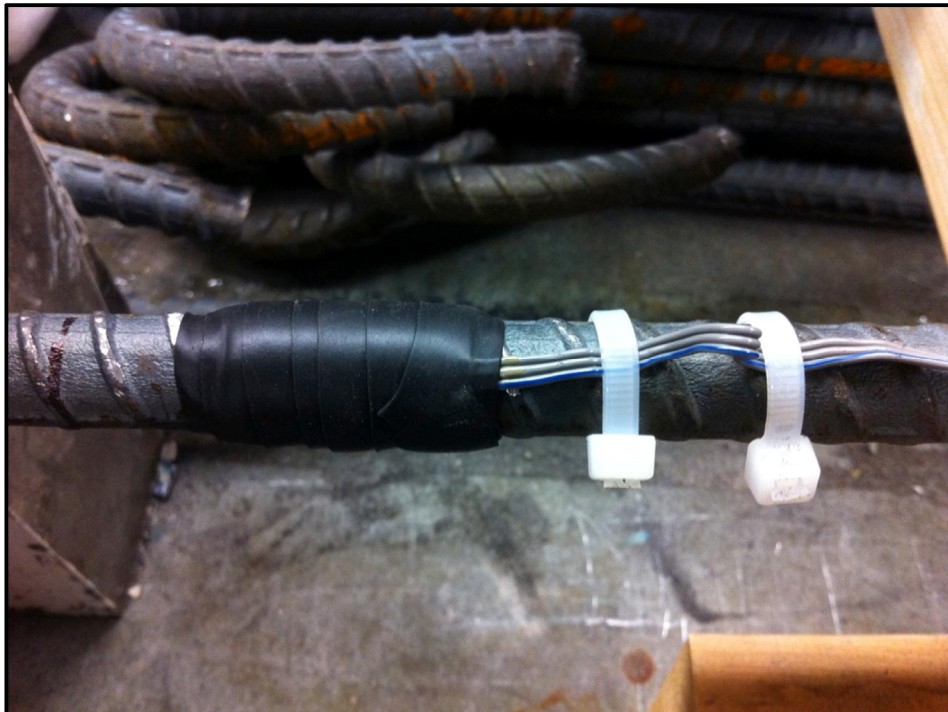
Figure 3-36 – ESG Installation With All Protective Coatings In Place (Typical)
