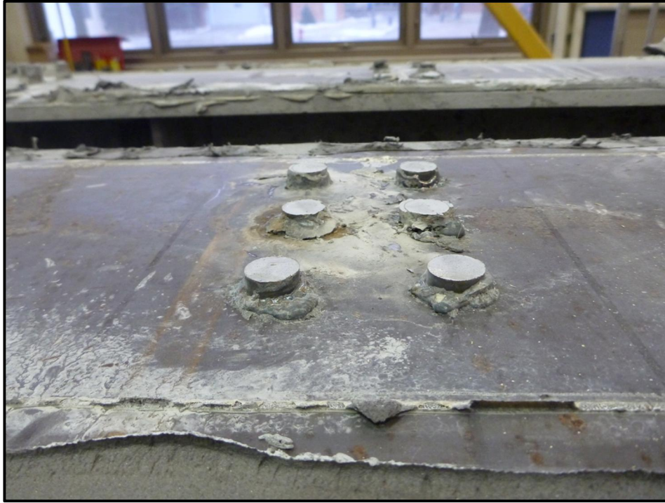
Figure 4-21 – Undamaged Shear Stud Cluster Far From Loading Point (Test #2)
