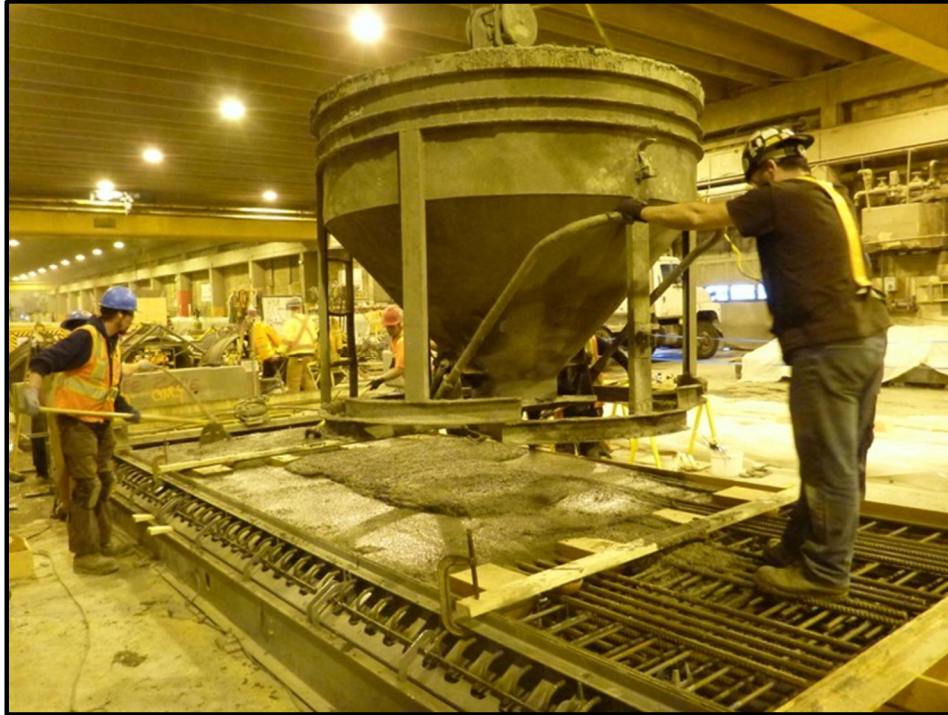
Figure 3-11 – Casting of PPCP Using Crane Hoisted Hopper
