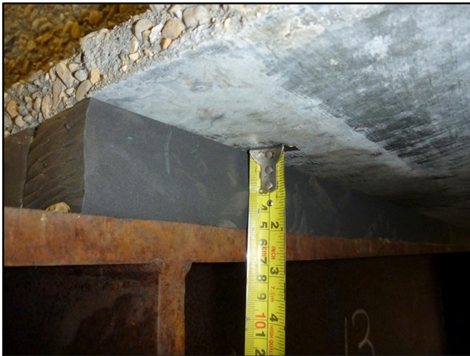
Figure 3-15 – EVA Foam Haunch Formwork Compressed from 75 mm to 50 mm After Panel Placement
