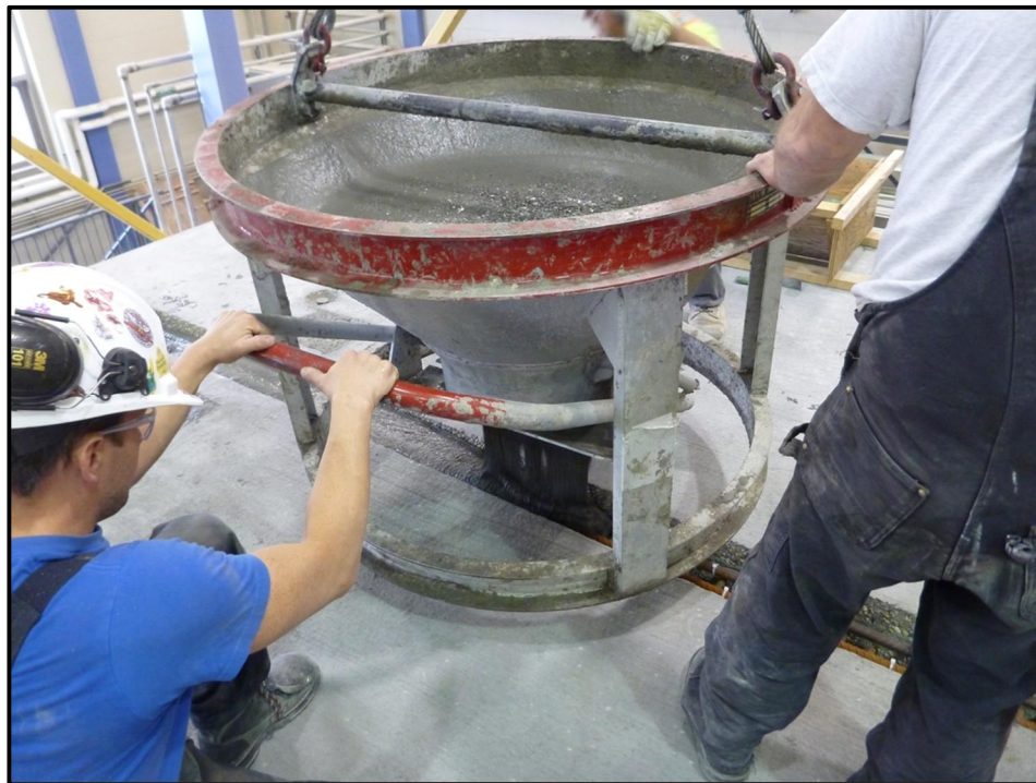
Figure 3-26 – Filling of Transverse Joint
