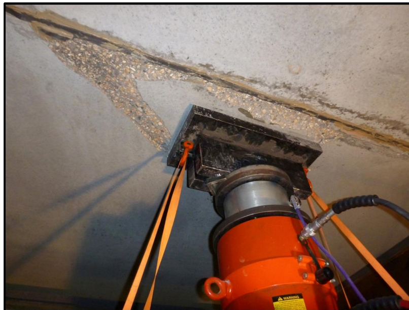
Figure 4-48 – Punching Shear Failure on Deck Soffit (Test #4)
