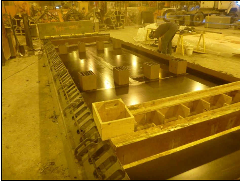
Figure 3-8 – Steel PPCP Formwork
