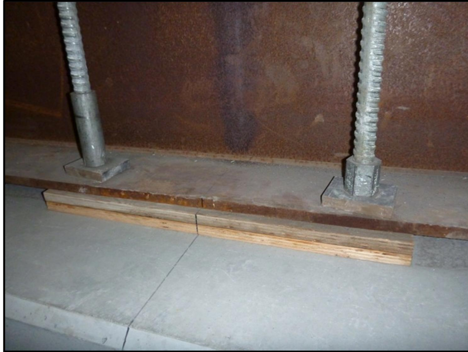
Figure 3-30 – Test Specimen Tie-downs on Exterior of Girders
