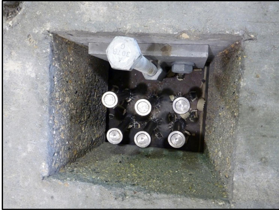
Figure 3-17 – Shear Studs Installed in Pockets Using Shear Stud Gun After PPCP Placement (TS1)
