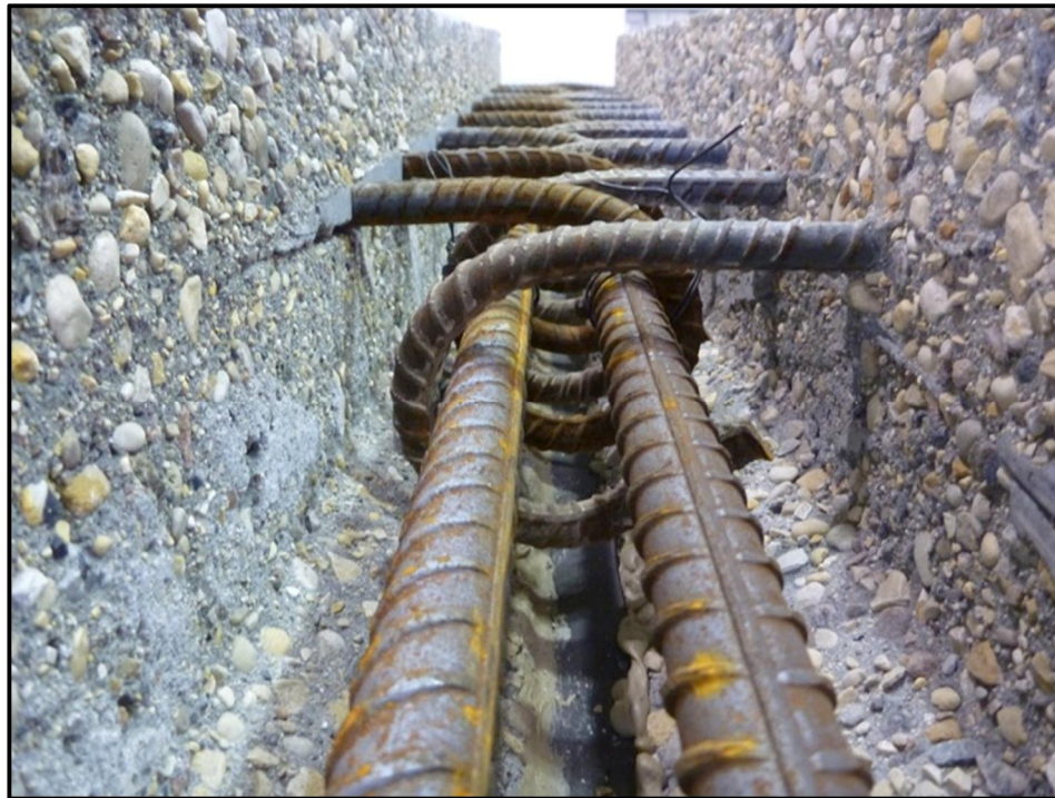
Figure 3-24 – Typical Reinforcing Steel within Transverse Joint (Two 25M Bars Across Top of Hooked Bars Not Shown)
