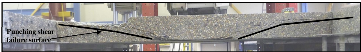
Figure 4-53 – Punching Shear Failure of Test Specimen #1 (Cut at Centerline of Panel/Loading Point)
