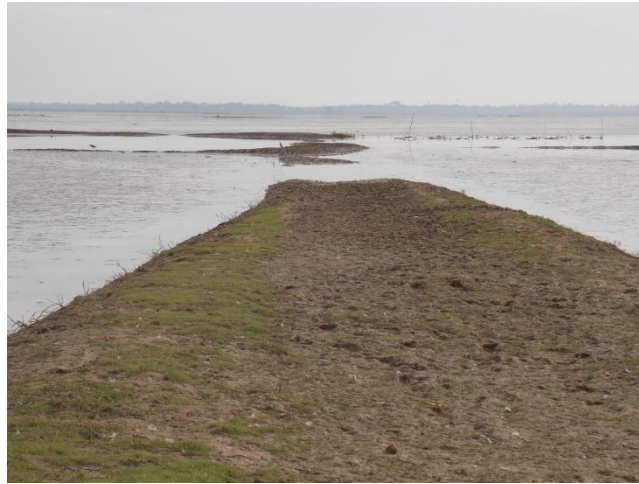
Plate 4.5: Image of a partially damaged embankment inside the haor
