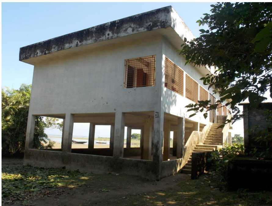
Plate 3.2: Image of a multipurpose flood shelter
