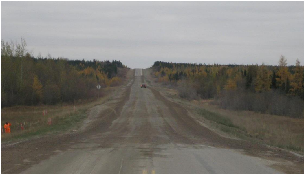
Figure 2: Unstable section of PR 391 in northern Manitoba (courtesy of Batenipour, 2014).
