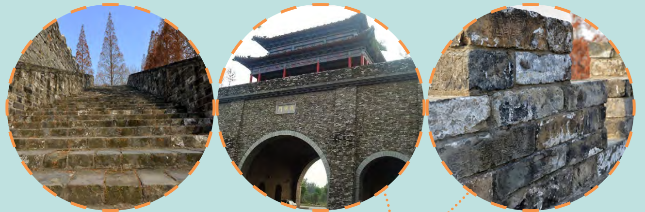
Figure 6.11 - Views of ancient wall in Nanjing.
