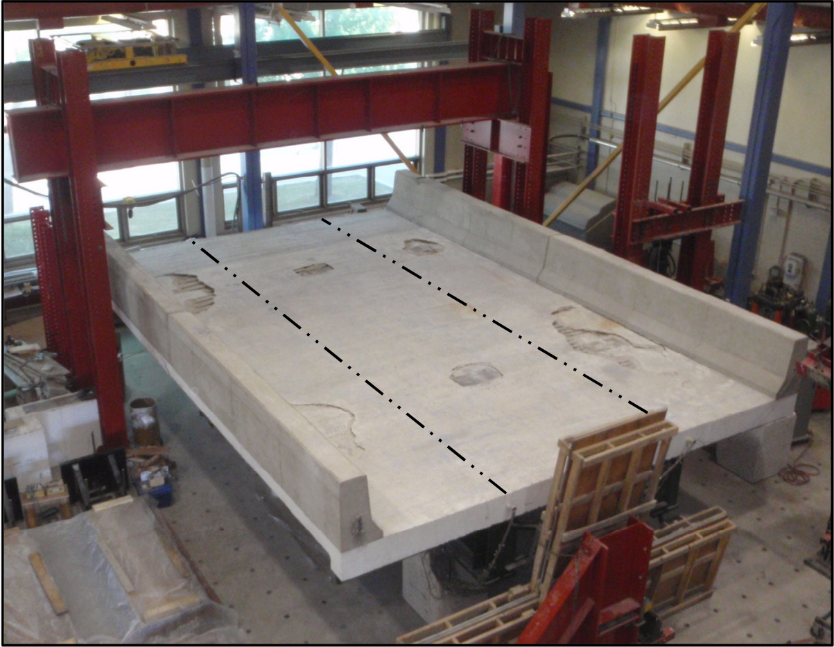
Figure 4-78: Photograph of the entire experimental bridge deck slab illustrating punching shear failures of the cantilever sections
