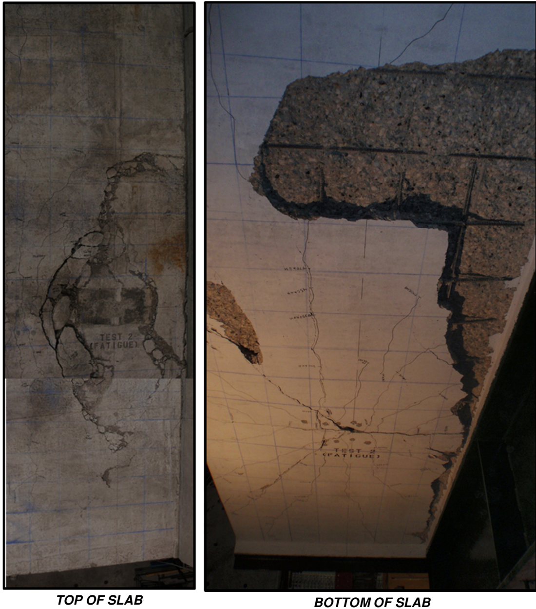
Figure 4-58: Photograph illustrating top and bottom crack patterns for the cantilever section with steel reinforcement subjected to fatigue cyclic loading
