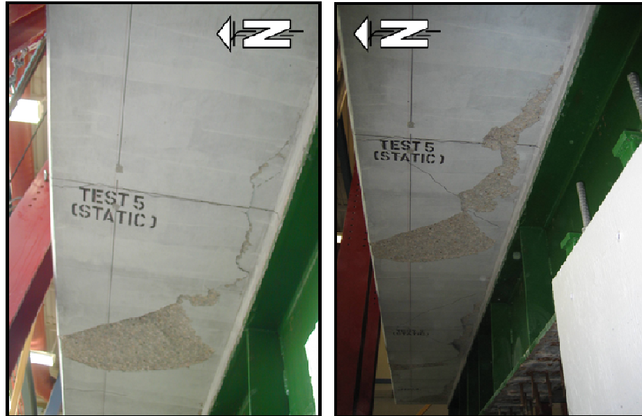
Figure 2-25(b): Bottom view of semi-circular punching type failure for cantilever section with top transverse GFRP reinforcement subjected to static monotonic loading (Klowak, 2007)
