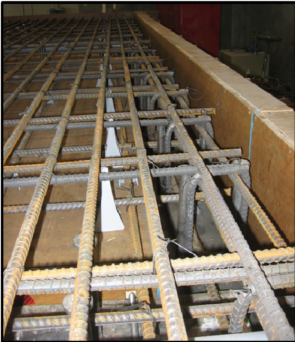
Figure 3-10: Photograph showing transverse steel bars and stirrups located in transverse edge beam
