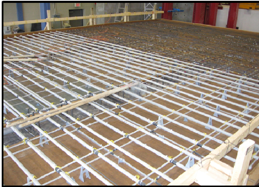
Figure 3-8: Photograph of internal GFRP and steel reinforcement prior to concrete placement
