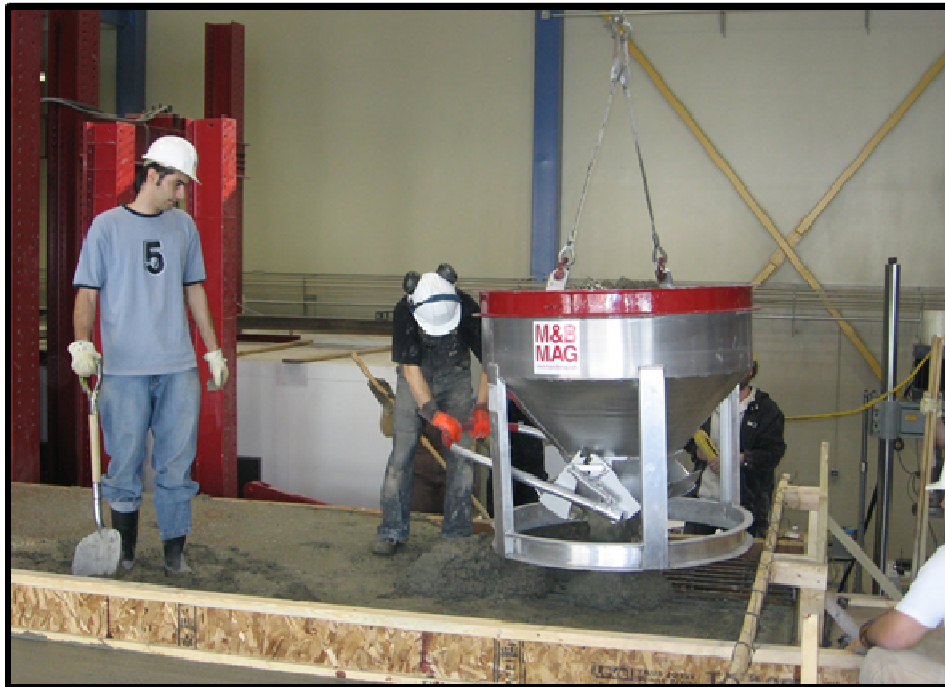
Figure 3-3: Photograph of concrete placement for experimental bridge deck slab
