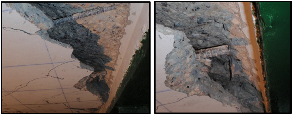
Figure 4-73: Photograph illustrating the rupture of the bottom transverse steel reinforcement for the cantilever with steel reinforcement subjected to a fatigue cyclic load
