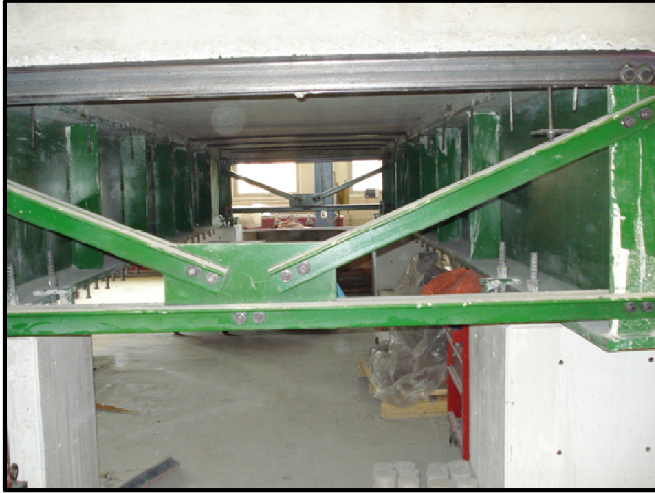
Figure 3-2(a): Photograph of end diaphragm
