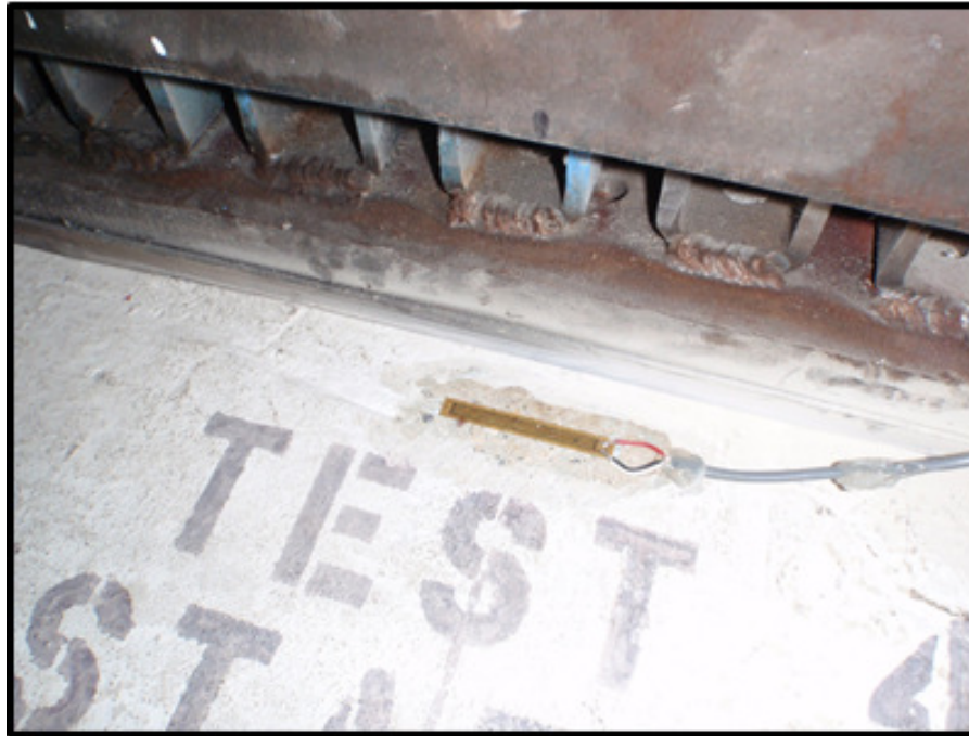
Figure 3-25: Photograph illustrating location of a concrete strain gauge placed in the transverse direction on the top surface of the cantilever slab overhang near the steel loading plate
