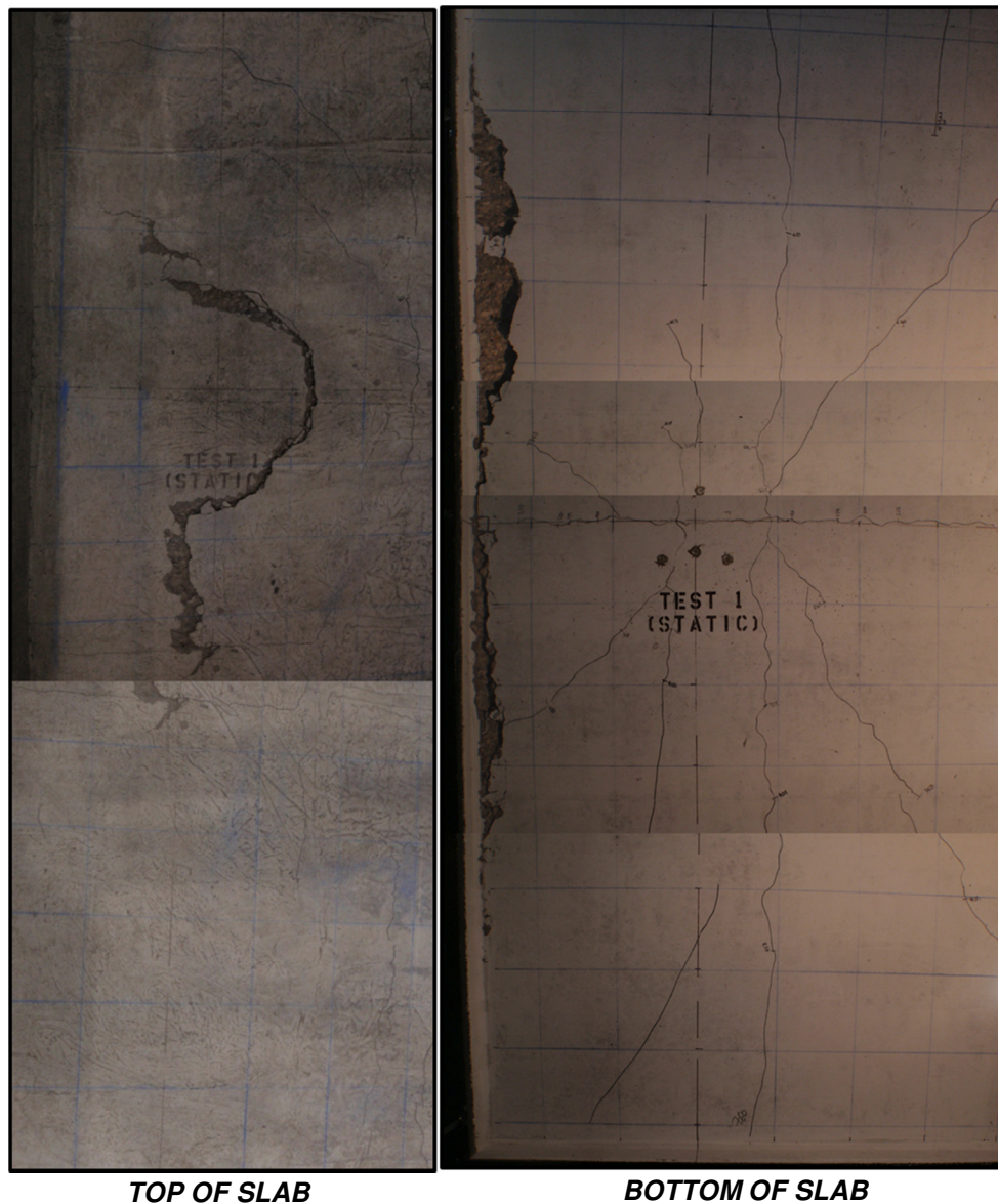
Figure 4-50: Photograph illustrating top and bottom crack patterns for the cantilever section with steel reinforcement subjected to static monotonic loading
