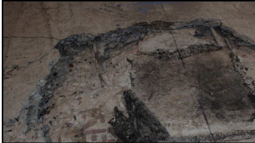
Figure 4-75: Photograph illustrating the top view of the pronounced punch cone for the cantilever with GFRP reinforcement (no rupture of top transverse GFRP reinforcing bars)
