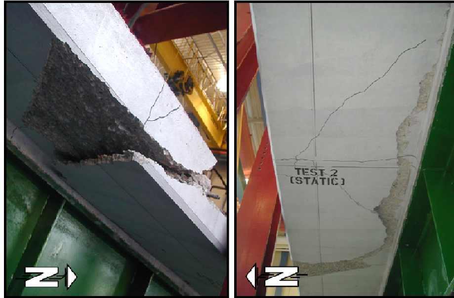
Figure 2-23(b): Bottom view of semi-circular punching type failure for the cantilever section with top transverse CFRP reinforcement subjected to static monotonic loading (Klowak, 2007)
