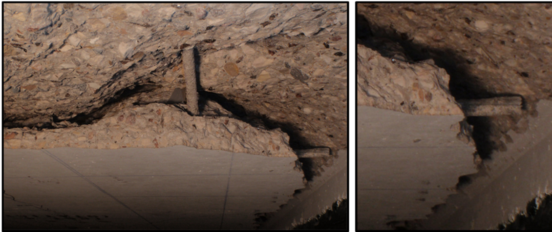
Figure 4-76: Photographs illustrating the rupture of the bottom transverse GFRP reinforcement for the cantilever with GFRP reinforcement subjected to a fatigue cyclic load
