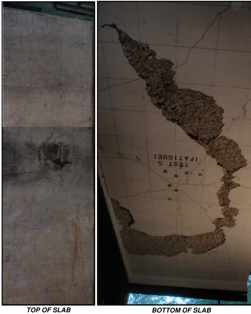
Figure 4-59: Photograph illustrating top and bottom crack patterns for the cantilever section with GFRP reinforcement subjected to fatigue cyclic loading
