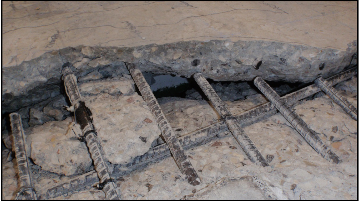
Figure 4-72: Photograph illustrating the rupture of the top transverse steel reinforcement for the cantilever with steel reinforcement subjected to a fatigue cyclic load
