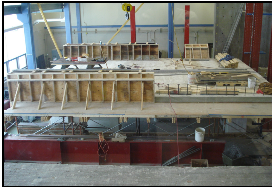
Figure 3-7: Photograph of traffic barrier wall construction
