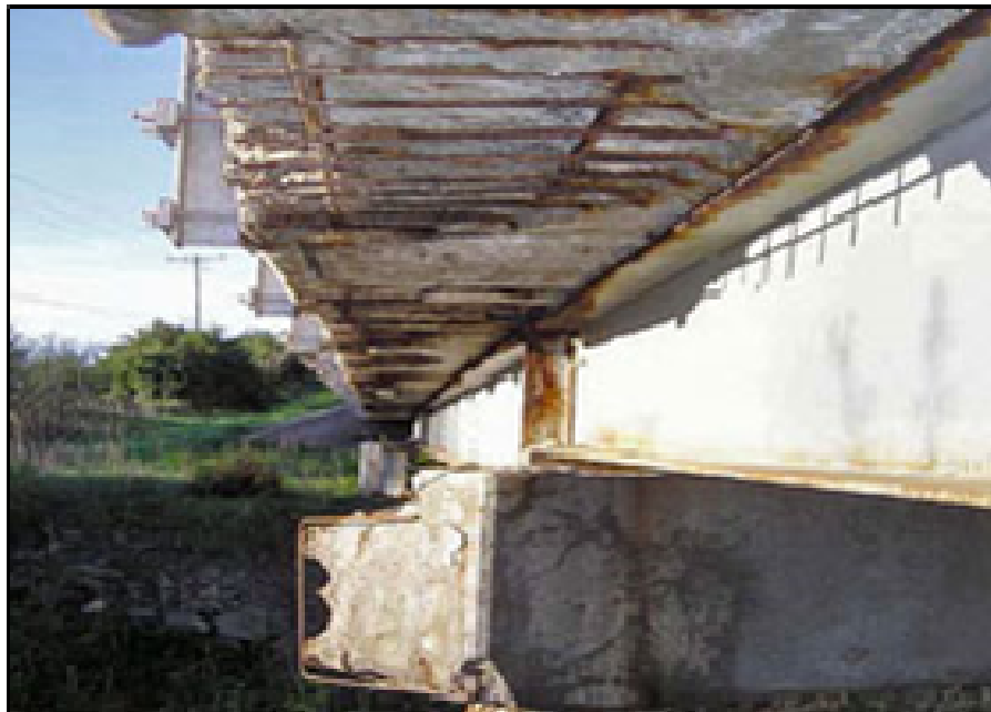
Figure 1-1(b): Deterioration caused by the corrosion of internal steel reinforcement in a cantilever overhang
