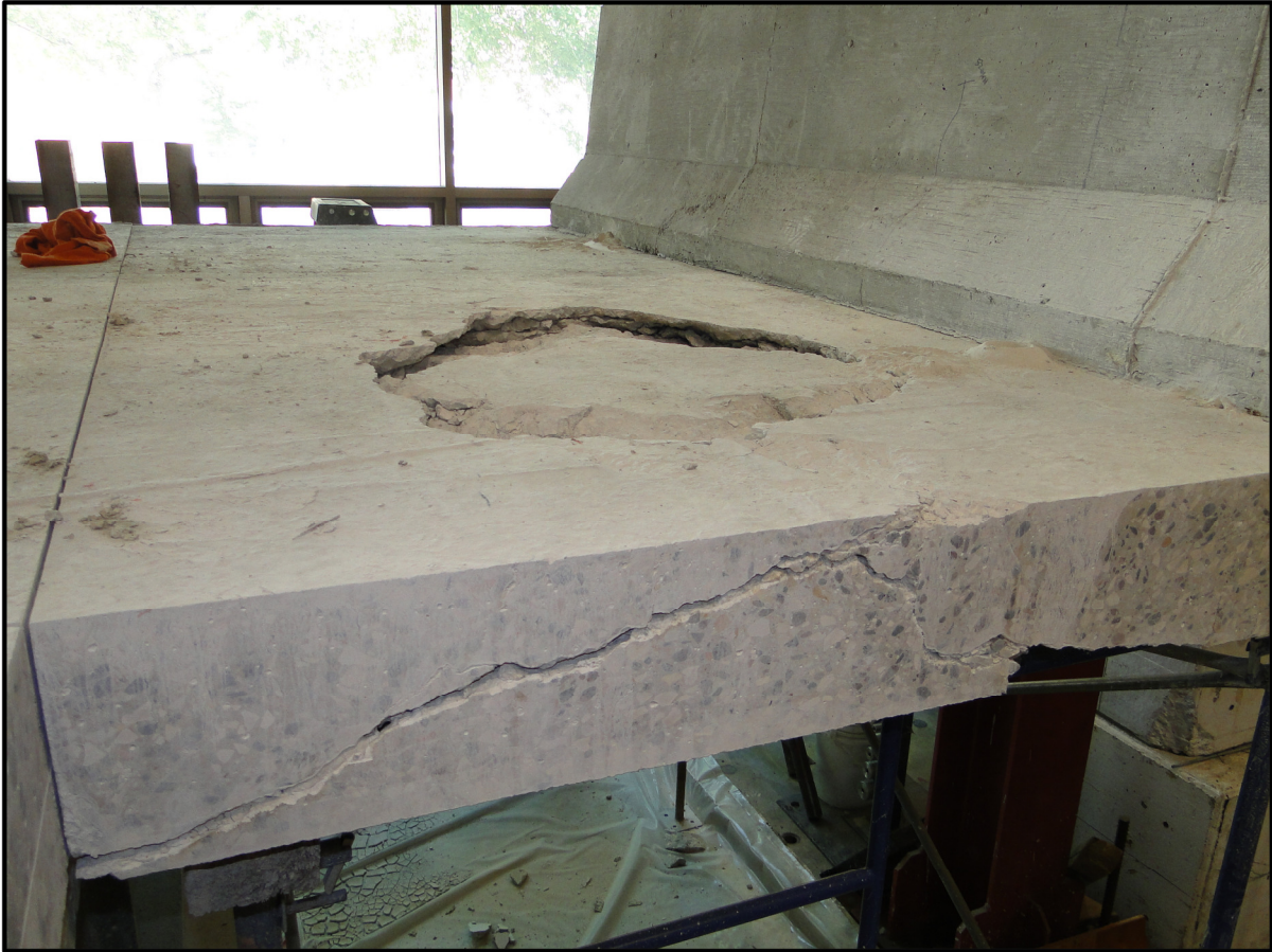
Figure 4-77: Photograph taken during demolition illustrating diagonal shear cracks and punch cone representative of punching shear failure for the cantilever with GFRP reinforcement subjected to a fatigue cyclic load
