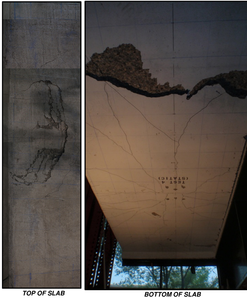
Figure 4-51: Photograph illustrating top and bottom crack patterns for the cantilever section with GFRP reinforcement subjected to static monotonic loading
