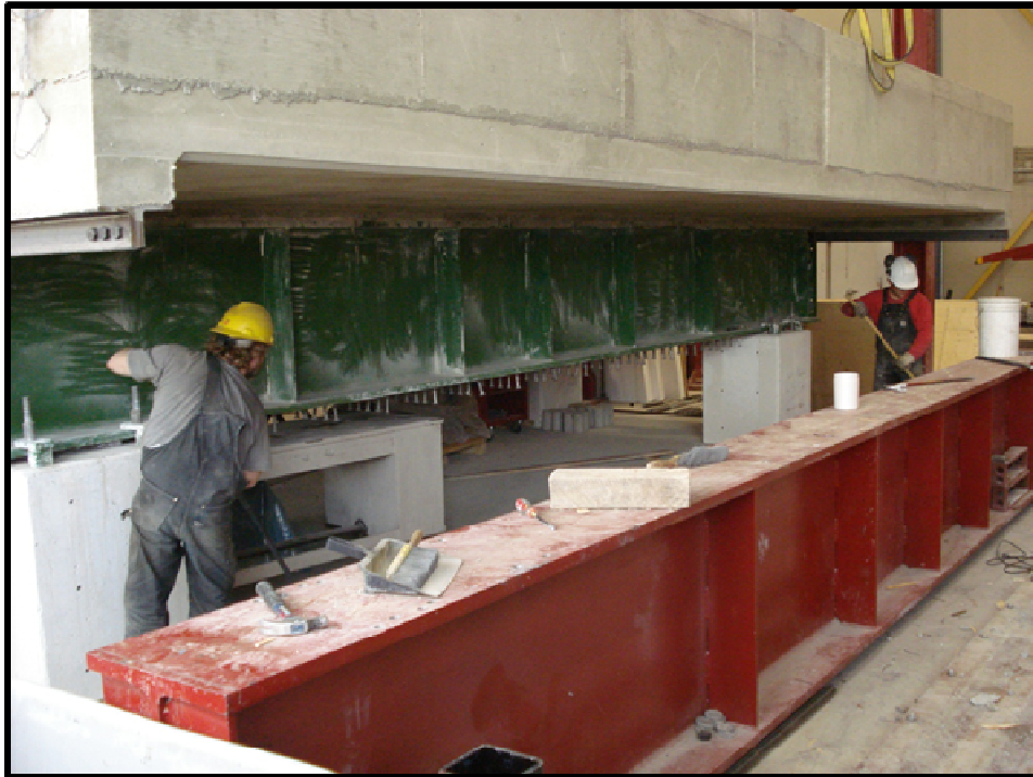
Figure 3-2(b): Photograph of steel girders after the removal of cantilever formwork
