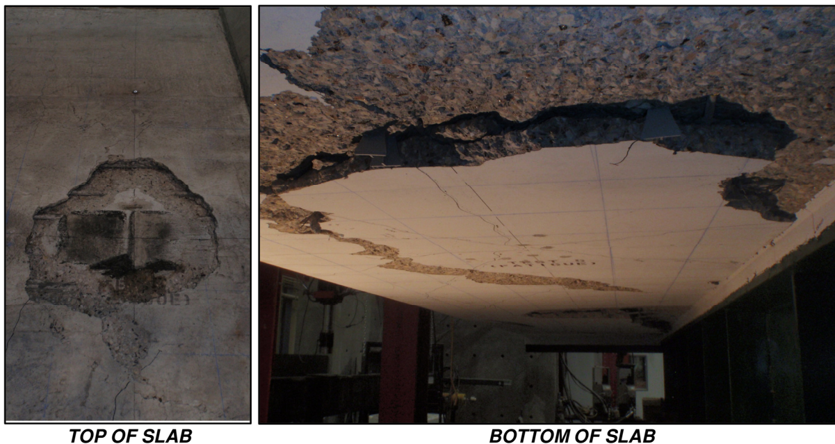
Figure 4-74: Photographs illustrating the top and bottom view of the pronounced punch cone for the cantilever with GFRP reinforcement
