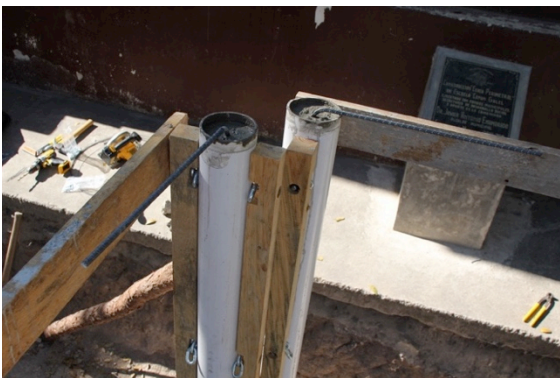
Figure I - 6: Concrete Filled PVC Tubes
