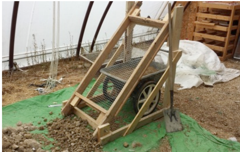
Figure 9: Sieving Earth With 1" Square Mesh Screen
