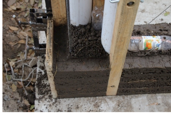
Figure I - 9: Rammed Adobe in Corner
