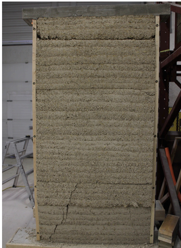
Figure 43: Racking Failure Wall 3
