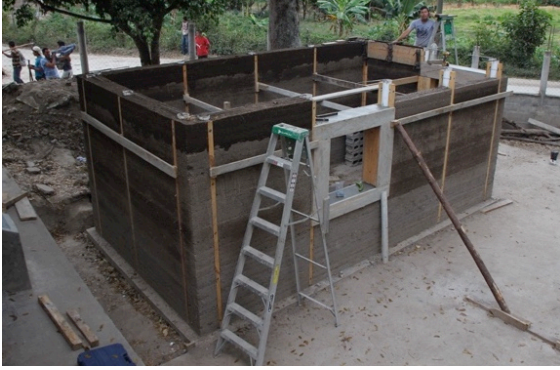
Figure I - 14: Last Infill Layer
