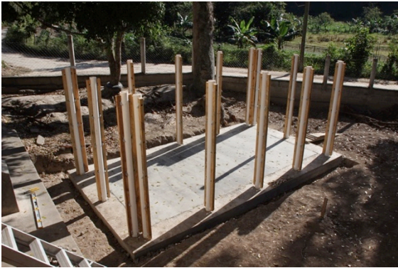
Figure I - 4: Setting the Columns
