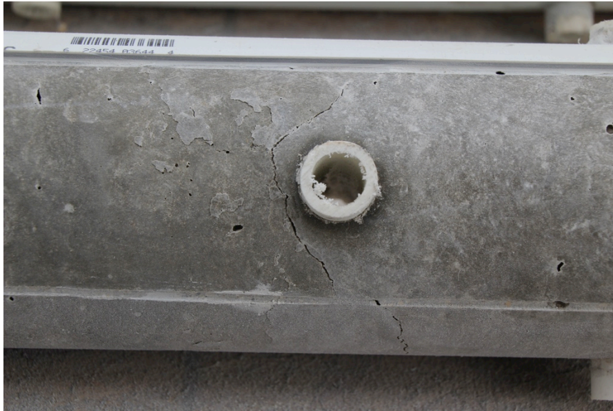
Figure 39: CFPT Hairline Crack @ 13 mm (1/2") PVC Insert Location
