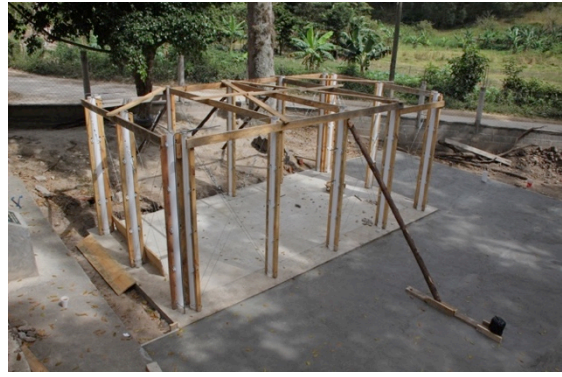
Figure I - 5: Bracing the Columns
