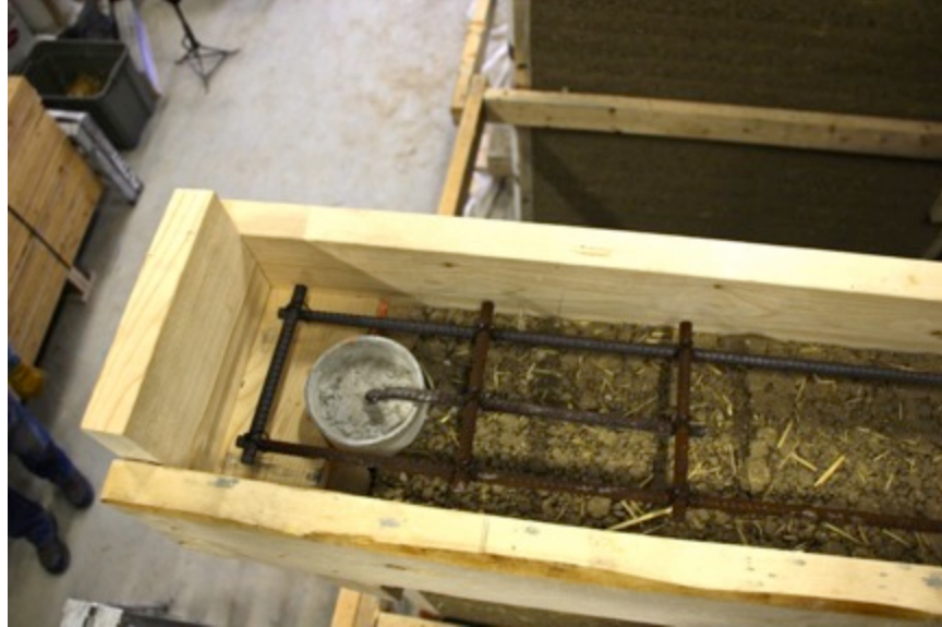
Figure 20: Bond Beam Formwork and Rebar
