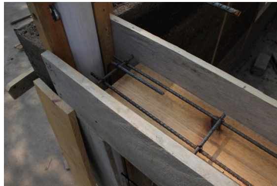
Figure I - 13: Door Formwork & Rebar
