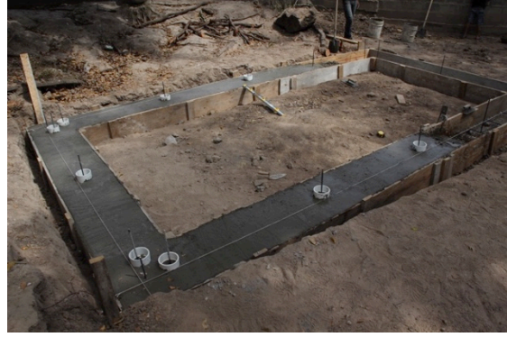
Figure I - 3: Concrete Footing
