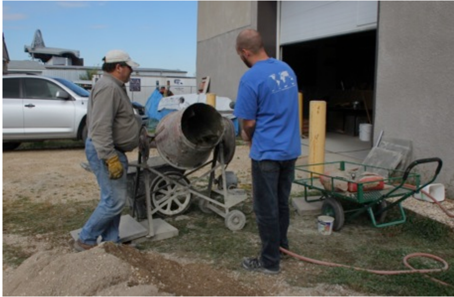
Figure 5: Mixing Concrete with Electric Blade Mixer
