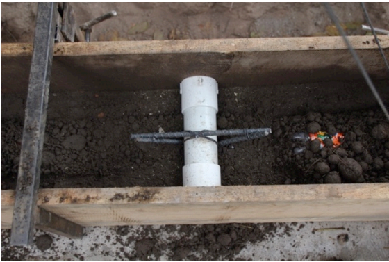
Figure I - 10: PVC Drain Pipe Embedment
