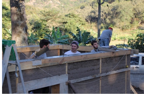
Figure I - 15: Concrete Bond Beam
