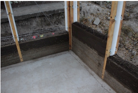
Figure I - 12: Start of Second Layer & Barbed Wire
