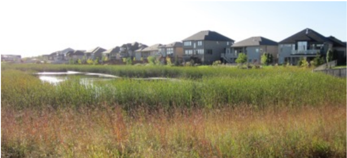
Figure 4: Mature naturalised retention pond in the Royal wood neighbourhood development in Winnipeg, Manitoba. (Photo by author, 2009.)
