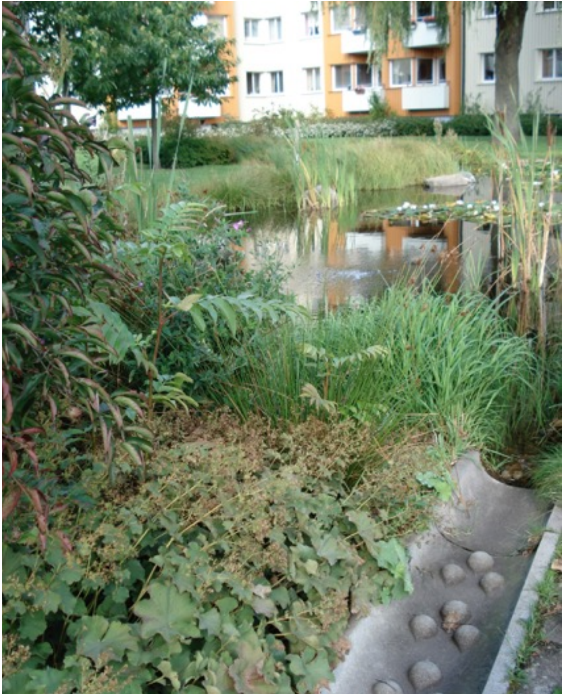
Figure 2: Wetland retention area and stormwater channel in Augustenborg, a densely developed 1950s social housing project in Malmö, Sweden. Augustenborg was renovated in 1999-2000 and retrofits redirect approximately 70% of total stormwater flows away from the local sewer system using stormwater channels (pictured above), wetland retention areas, and green roofs (Villarreal, Semadeni-Davies & Bengtsson, 2004). (Photo by author, 2008.)
