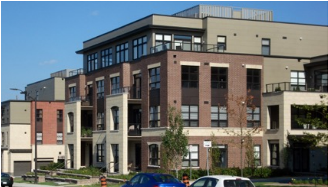
Figure 7: Rainwater capture in the Ampersand neighbourhood development in Ottawa, Ontario. (Photo by R. Kotak, 2013, used with permission.)
