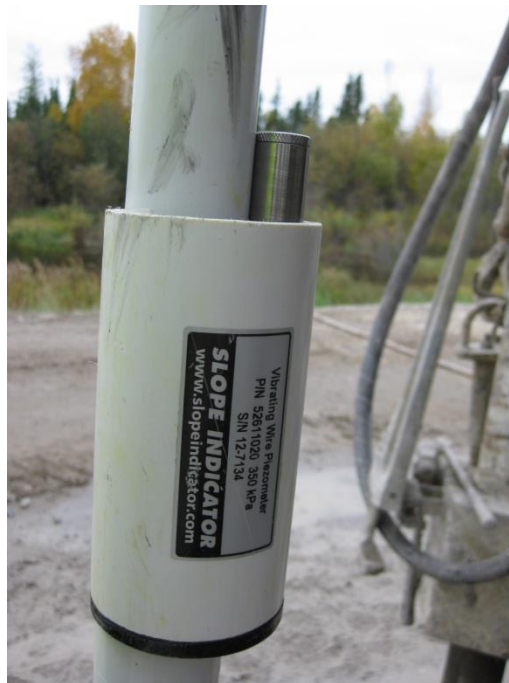
Figure 4.4: Multilevel Vibrating Wire Piezometer installed in the shoulder. September 24, 2012.
