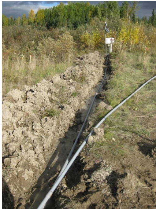
Figure 4.18: Trench dug to protect cables in the PVC pipe armoring to the DA Boxes. September 15, 2012.
