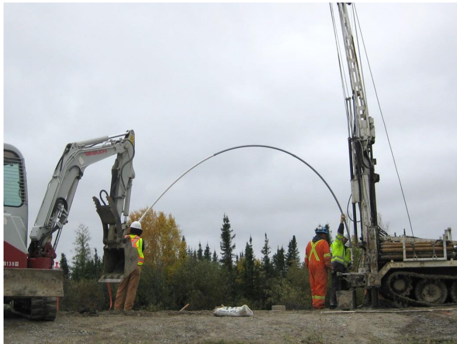
Figure 4.8: Installation of the Multilevel Vibrating Wire Piezometer at the Centreline on September 24, 2012.
