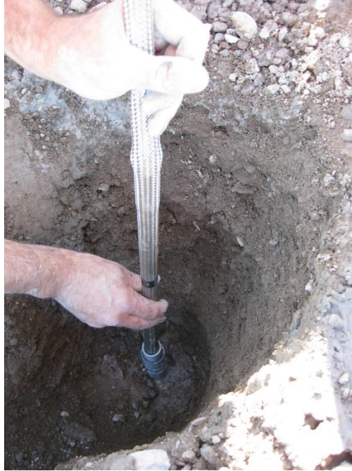
Figure 4.9: Installation of the vertical SAA at the shoulder into PVC pipe on September 15, 2012.
