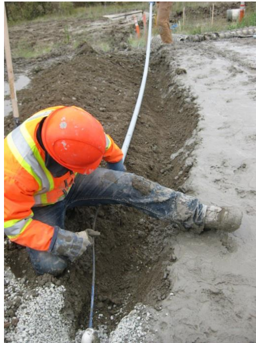
Figure 4.14: Pulling the thermistor cable through PVC pipe for extra protection as it runs from the centreline to the DA box. September 13, 2012.
