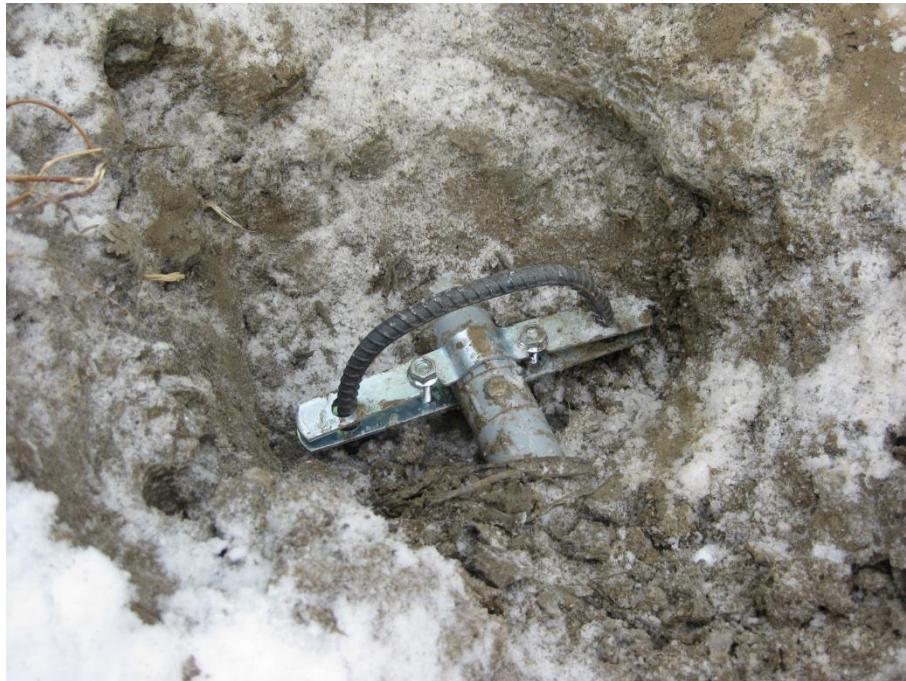
Figure 4.12: Installation of foot-long U-shaped piece of rebar as an anchor for the horizontal SAA installed at the toe. December 1, 2012.
