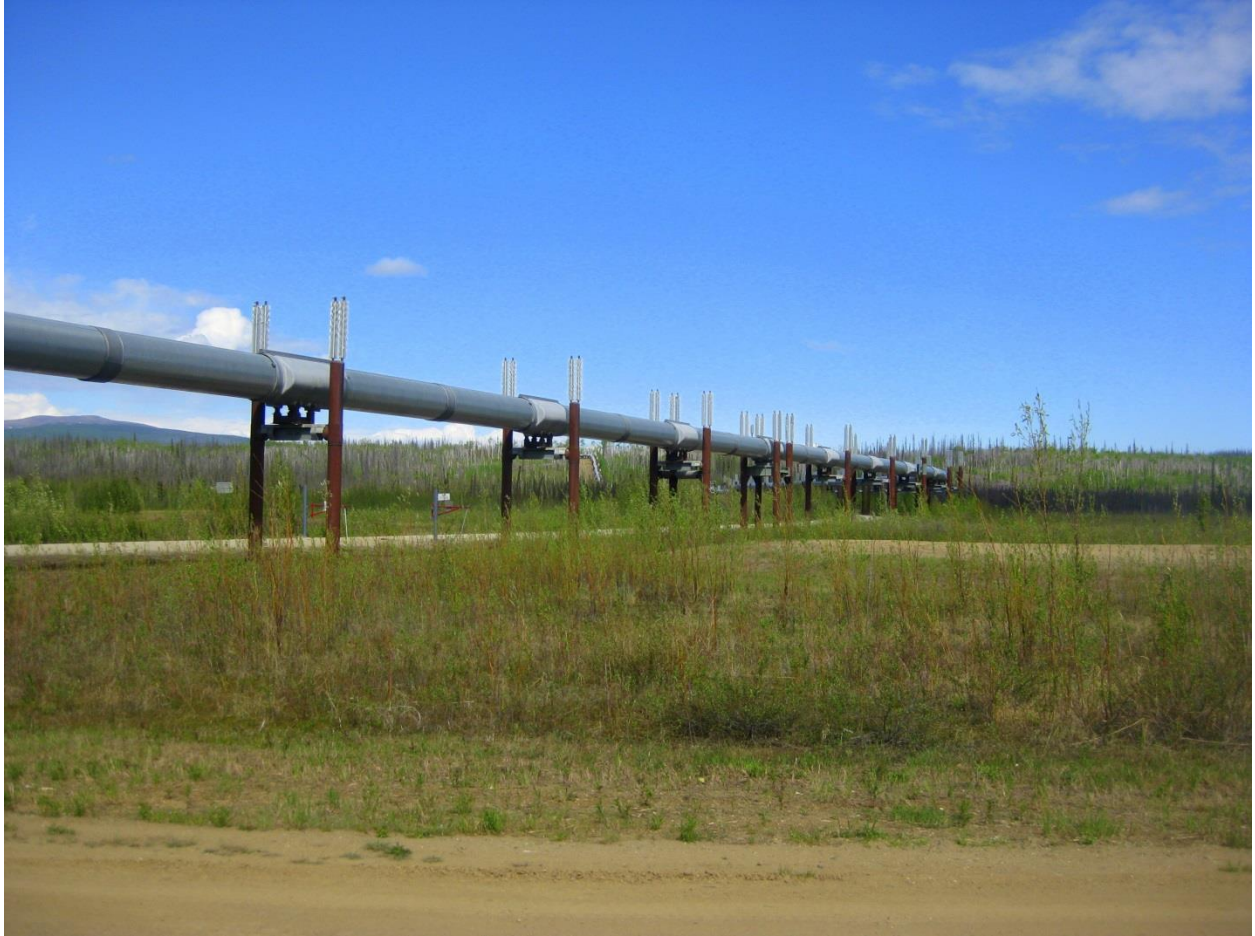
Figure 2.9: Thermopiles used as a passive heat extraction device for the Alaska pipeline near the Yukon River
