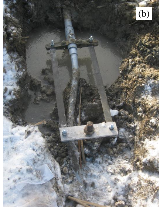
Figure 4.13: (a) Installation of 8-foot (2.4 m) long ground anchor to (b) complement the existing anchor for the horizontal SAA installed at the toe on November 14, 2013.
