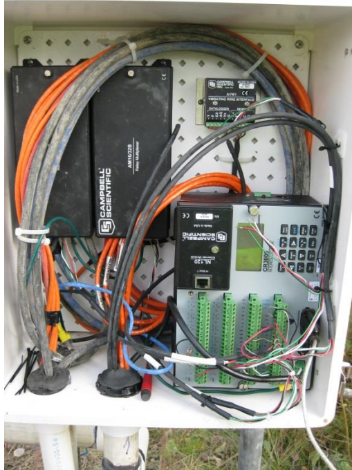
Figure 4.21: Housing containing (Clockwise from top left) multiplexers for the thermistors and VW piezometers (AM16/32B), vibrating wire Interface, CR3000 Micrologger, and Ethernet Module (middle on CR3000). September 16, 2012.
