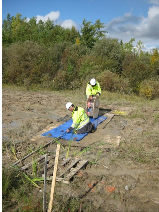
Figure 4.11: Installation of the horizontal SAA at the toe into PVC pipe on September 13, 2012.
