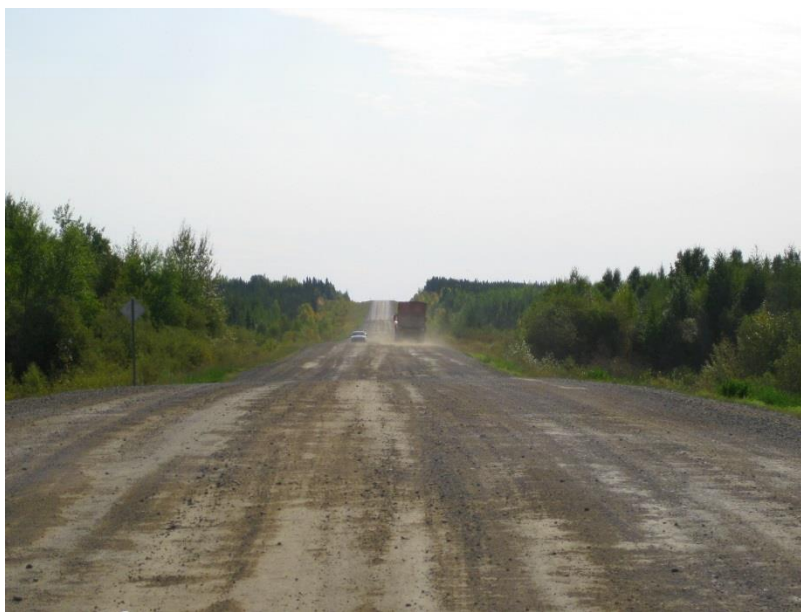
Figure 3.4: PR 391 Project Site. September 10, 2012.
