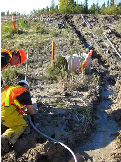
Figure 4.17: Additional armoring of horizontal SAA at the toe and view of the trench dug for the cables in the PVC pipes from the shoulder of the embankment. September 15, 2012.
