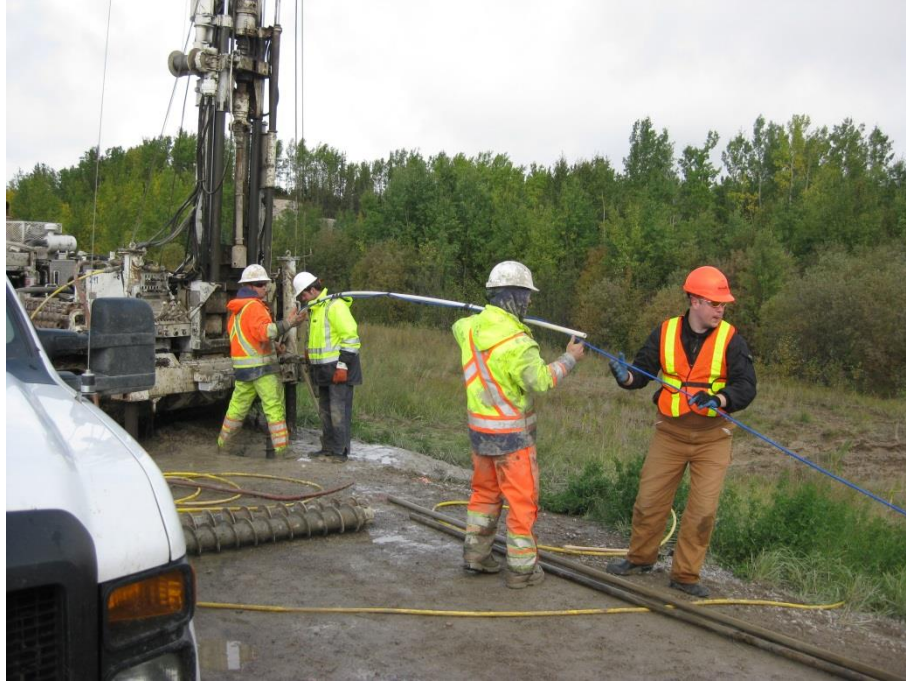
Figure 4.7: Installation of the 13-Point Thermistor 18m in length at the Shoulder on September 12, 2012.
