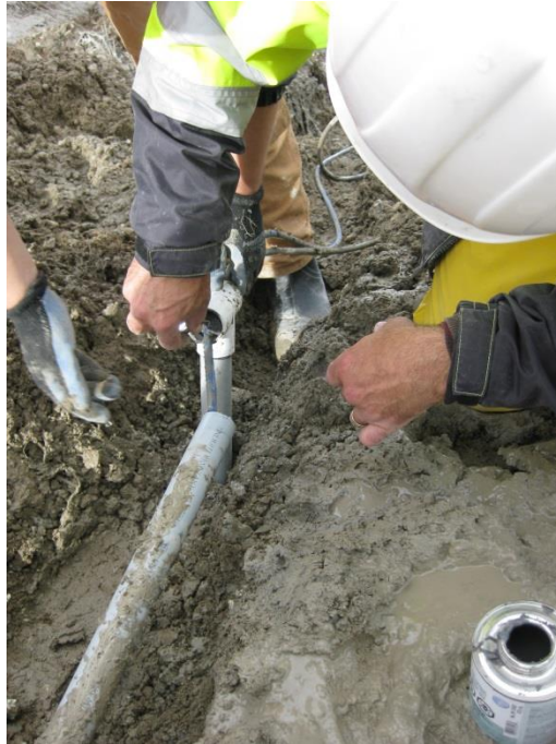
Figure 4.15: Gluing a connection for the PVC pipe protection of instrumentation cables at the shoulder. September 13, 2012.
