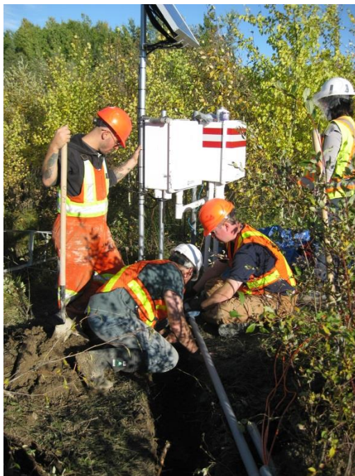
Figure 4.19: Fitting final connections of PVC pipe that contain the instrumentation cables to the DA boxes. September 14, 2012.
