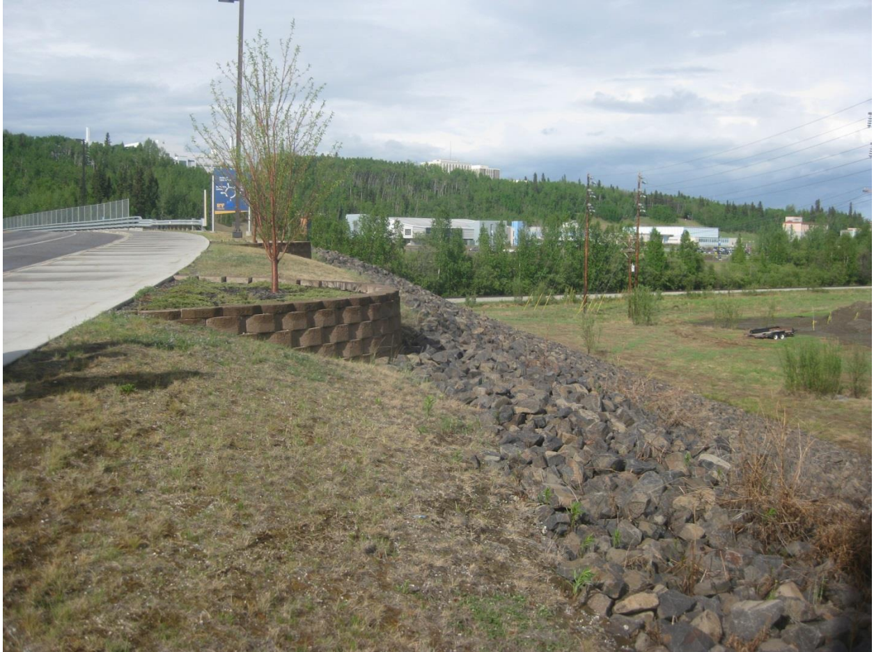
Figure 2.10: Air Convection Embankment used on the approach for the bridge over the Alaska Railroad on Thompson Drive in Fairbanks, Alaska.
