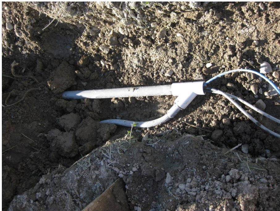
Figure 4.16: Instrumentation cable protection at the shoulder. September 15, 2012.
