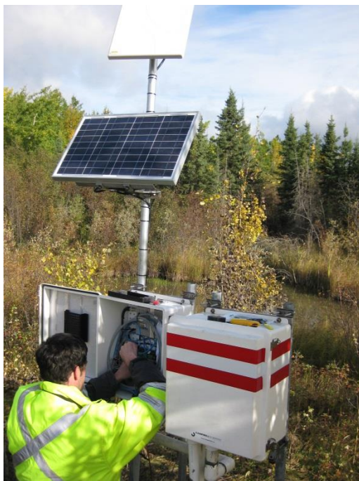
Figure 4.20: Wiring the instrumentation into the data acquisition system. Top: Satellite. Middle: Solar Panel. Bottom: Housing for Data Acquisition System. September 16, 2012.
