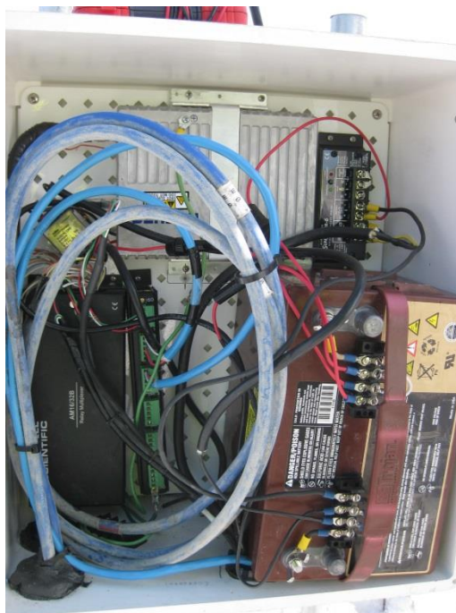
Figure 4.26: Housing contained (clockwise from top left) the relay switch, communication array, new solar regulator, new 15-volt AGM battery, and multiplexers. March 27, 2013
