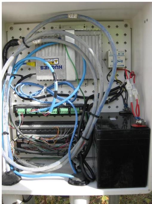
Figure 4.22: Original set up for left housing including (clockwise top left) communication array, original solar regulator, original battery, and multiplexers (SAA multiplexer on top and AM16/32B Multiplexer on bottom). September 16, 2012.
