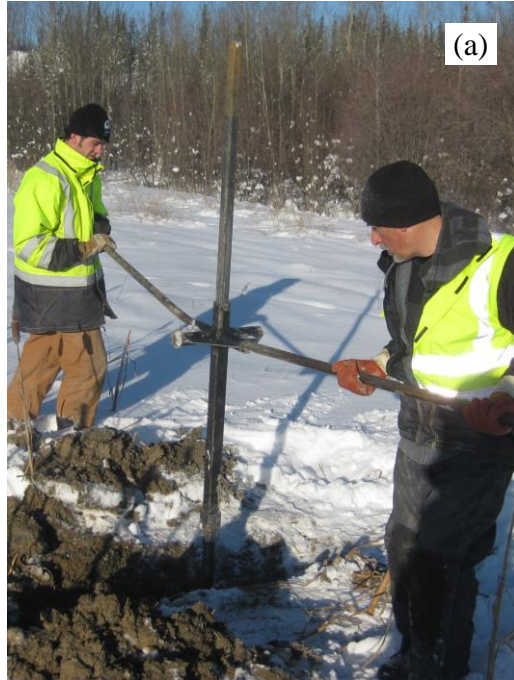
Figure 4.13: (a) Installation of 8-foot (2.4 m) long ground anchor to (b) complement the existing anchor for the horizontal SAA installed at the toe on November 14, 2013.
