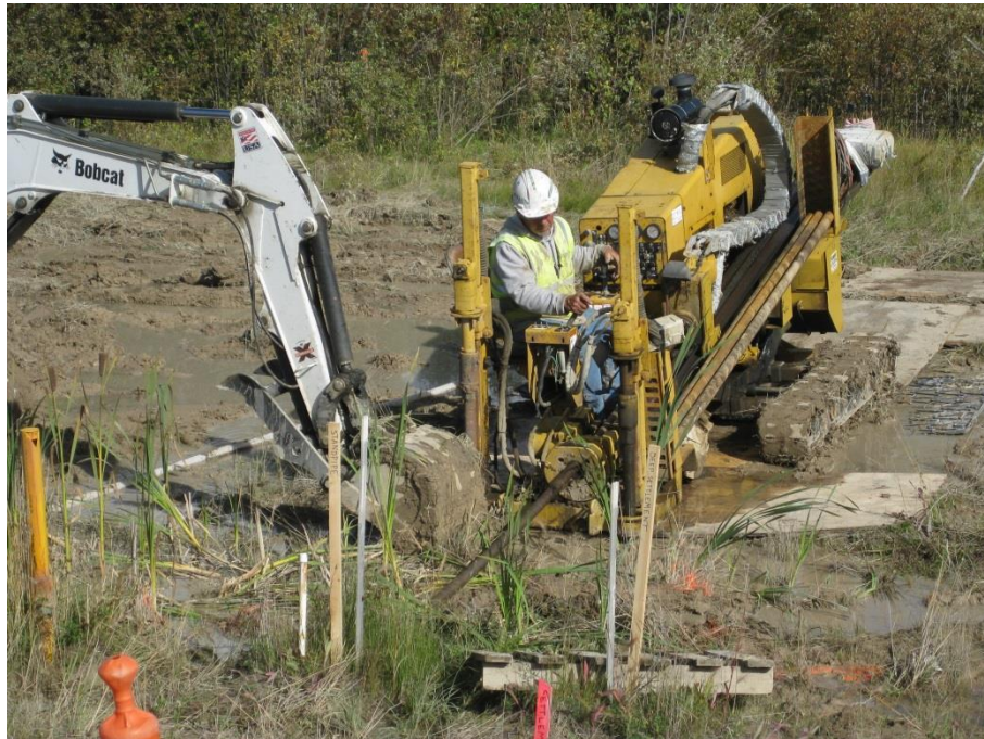
Figure 4.10: Horizontal drilling on September 13, 2012 at the toe of the embankment for the horizontal SAA installation.
