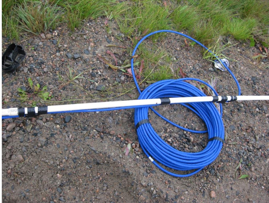
Figure 4.3: RST Thermistor ready for installation into the shoulder. Electrical tape was used to secure the thermistor nodes to the PVC pipe. September 12, 2012.
