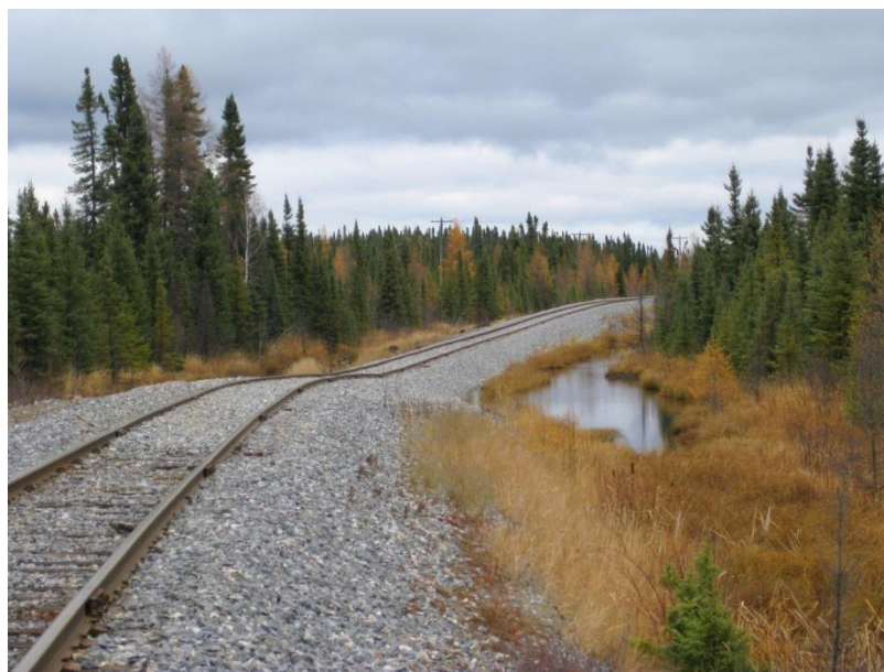
Figure 3.2: Settlement due to Permafrost Conditions on the Hudson Bay Railway north of Thompson. October 21, 2012.
