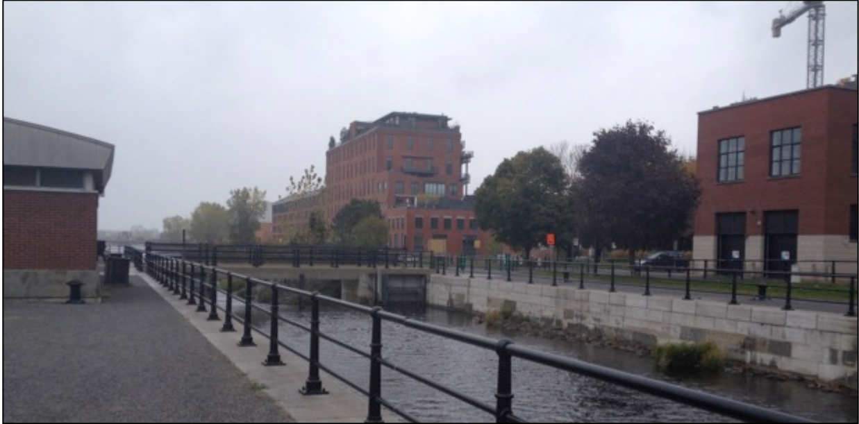
Figure 24: Lachine Canal facing southeast (Elias, 2014)
