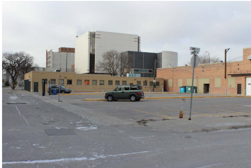
Figure 8: The intersection of James Avenue and Amy Street, an example of missing street curbs with the WDN.
