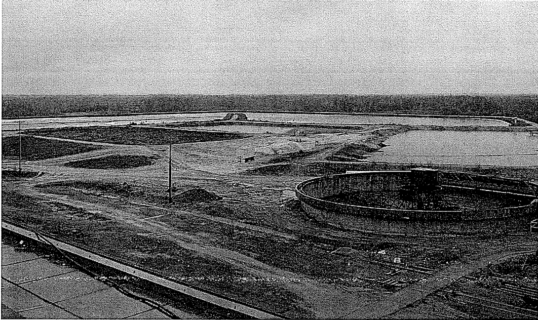
Image 4.3: Lagoon at Tolko Industries site just outside of The Pas
