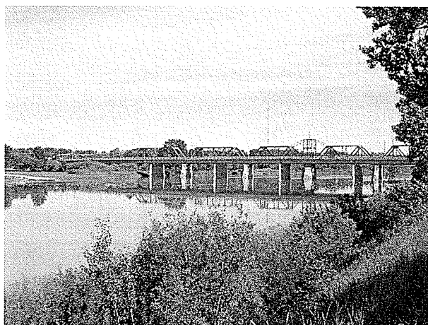
Image 4.5: Bridge linking The Pas and OCN
