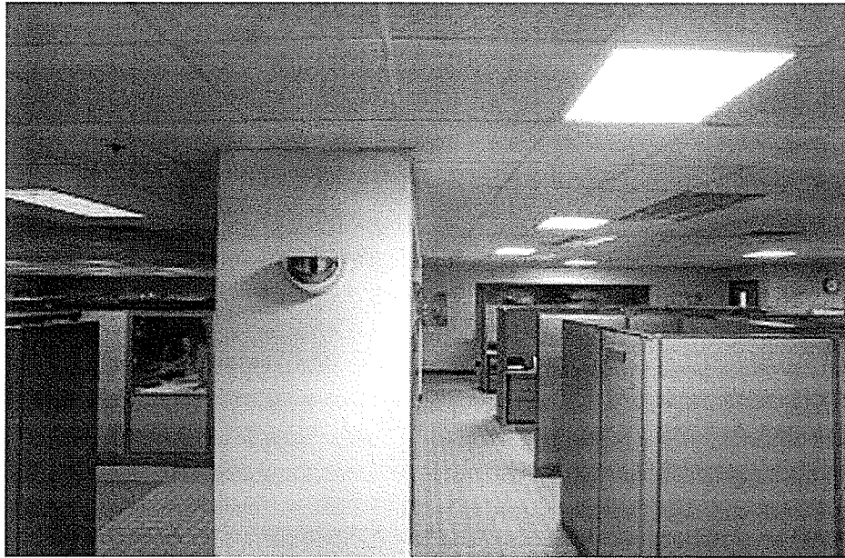
Figure 55. Office space illuminated by standard fluorescent lighting on left side of image, and Velux sun tunnel skylights on the right. Image property of Velux Canada.
