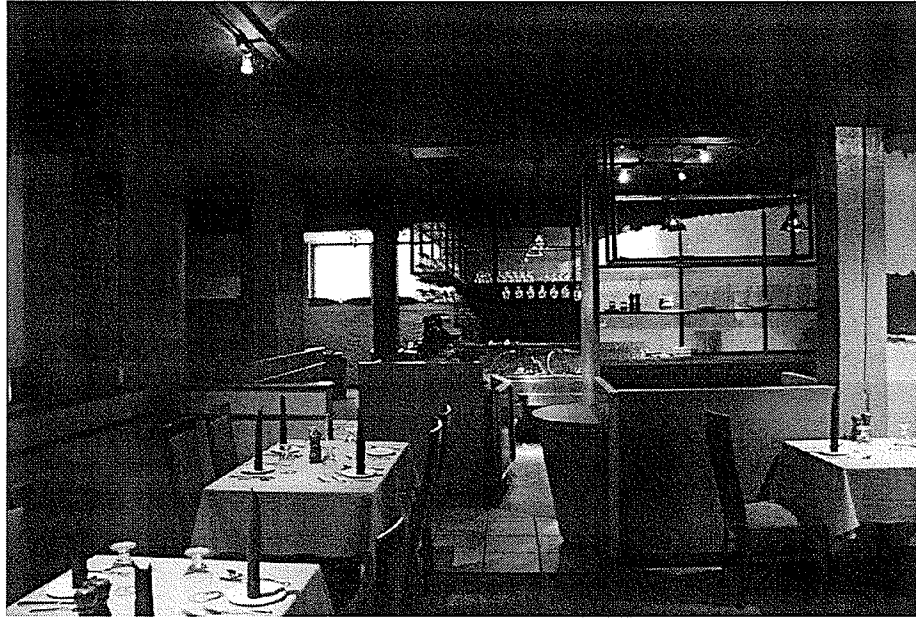
Figure 26. View of basement level restaurant — load-bearing timber posts are painted an olive green, which could be sandblasted before renovation begins.
