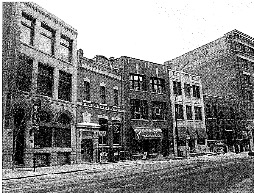
Figure 5. Adjacent buildings to 169 – 171 McDermot Avenue.
