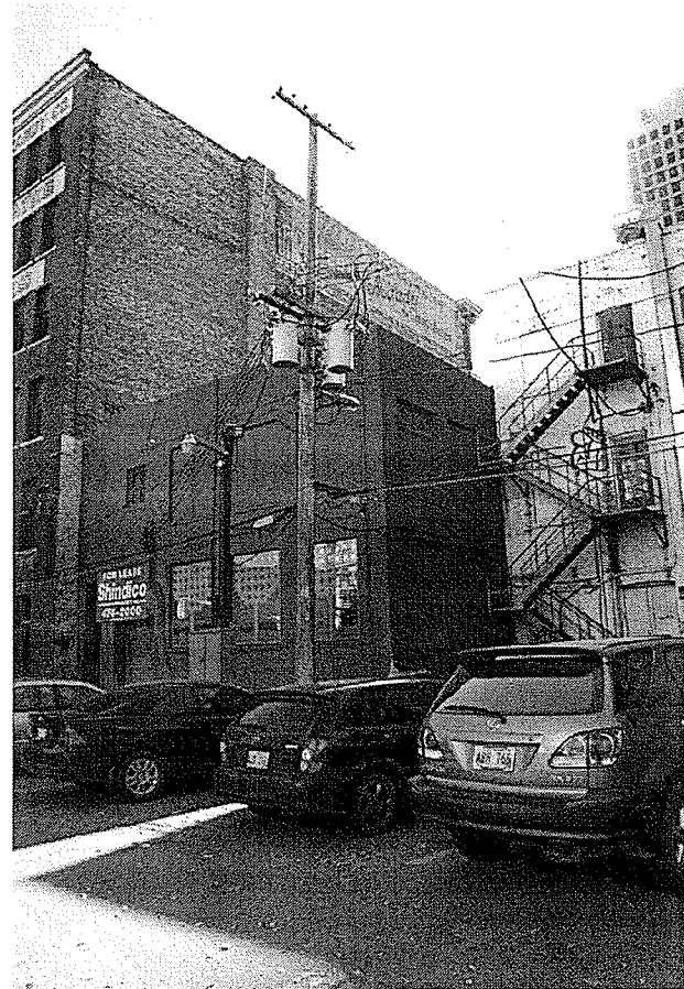
Figure 15. The north wall of 171 McDermot Avenue consists of large windows contributing to the vulnerability to south moving wind. Image shows diffused light on October 3, 2007, 1:36 pm.
