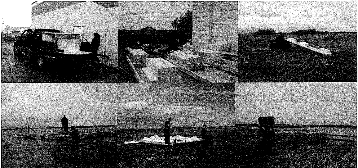
Figure 2 Construction of the enclosure and assembly in the marsh.
