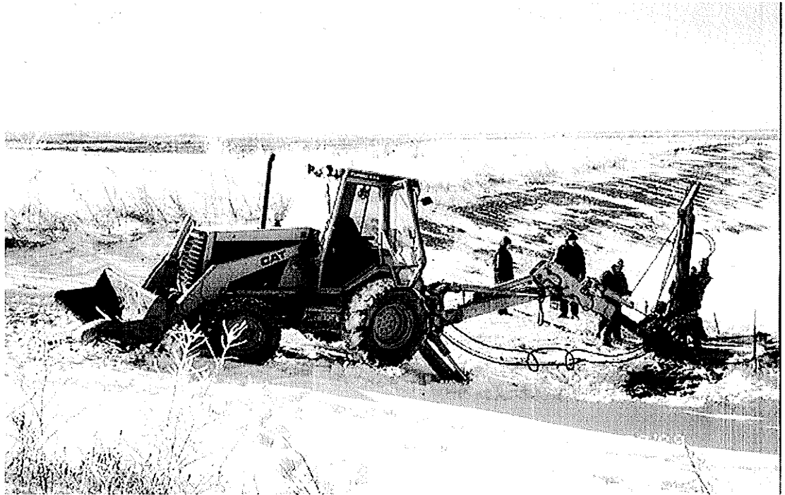
Figure 4.2 a: Backhoe-mounted Drill Rig
