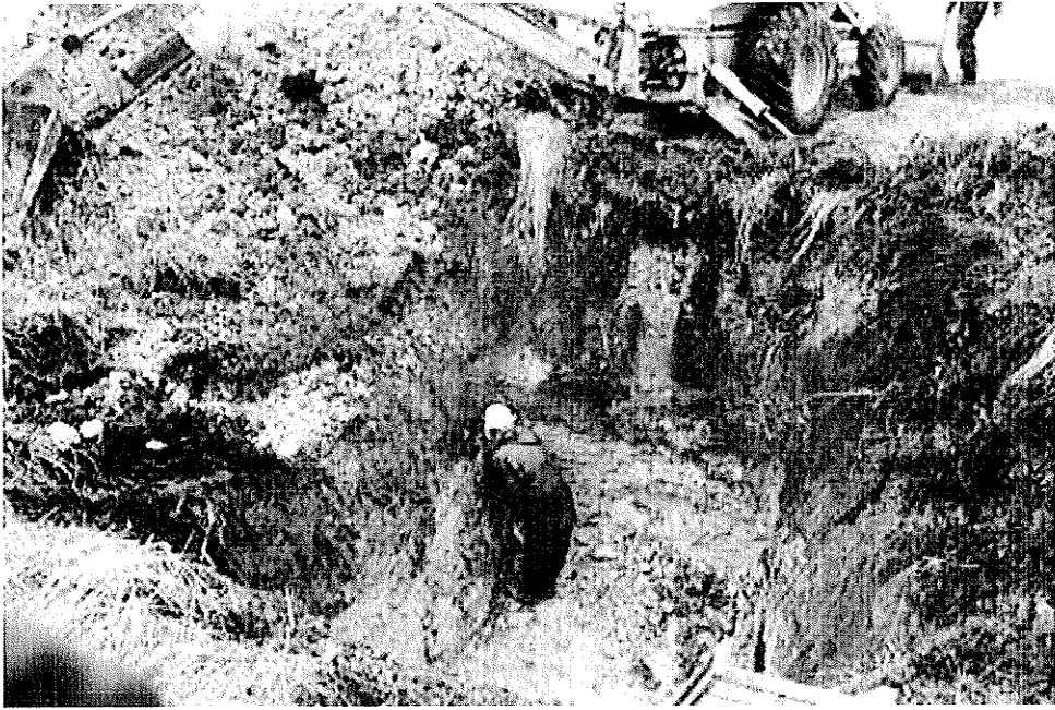
Figure 4.8 b: NC1 Test Pit
