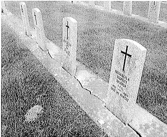
Figure 3. Severe longitudinal cracking.
