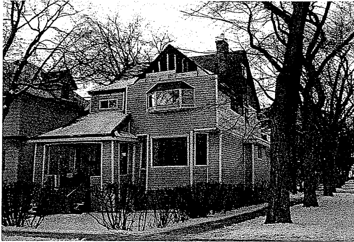
Figure 4.18 Character Home in McMillan under repair
