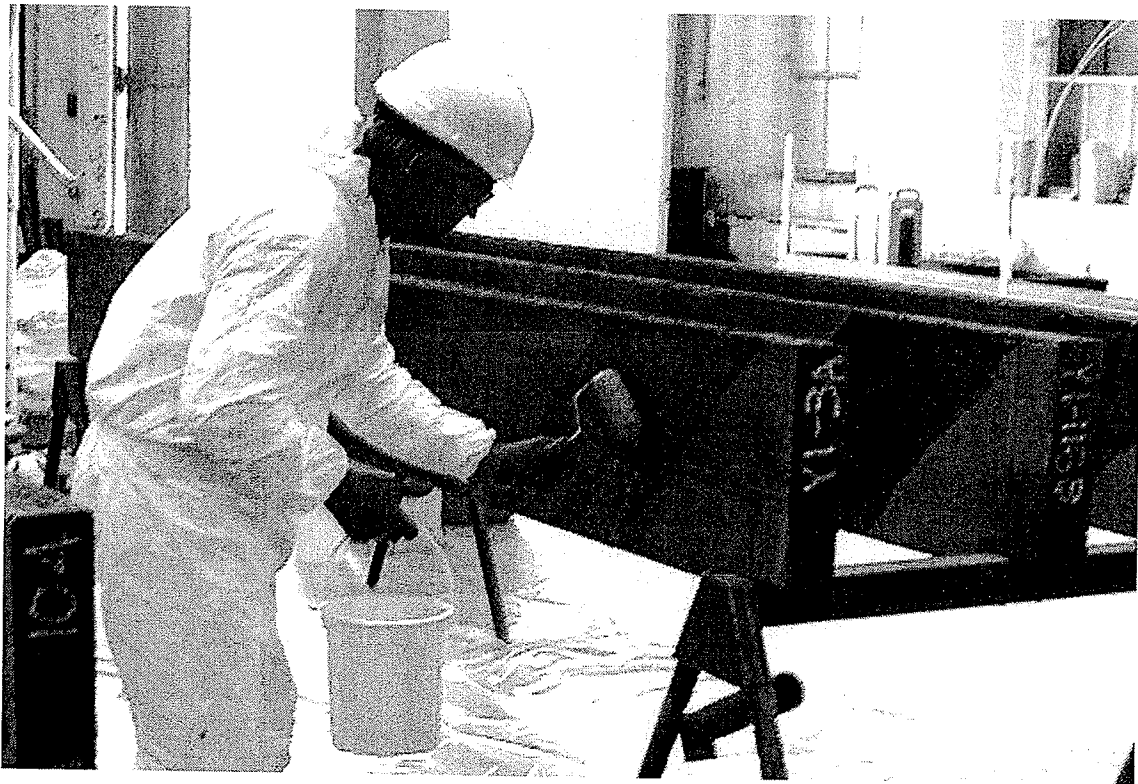
Figure 3.10 Applying primer
