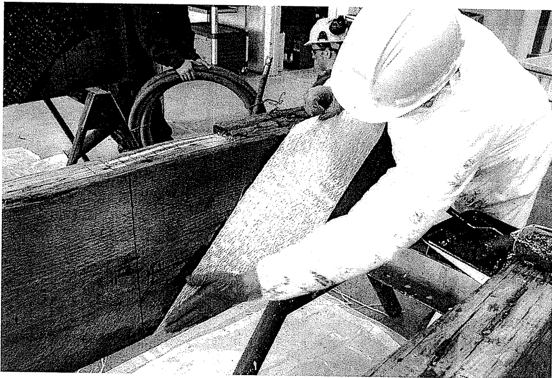
Figure 3.12 Placing GFRP sheet
