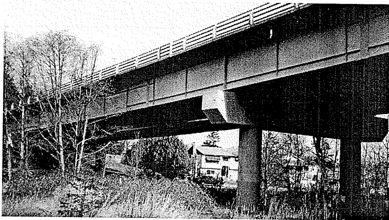
Figure 7: Portage Creek Bridge, Victoria, British Columbia, Canada
