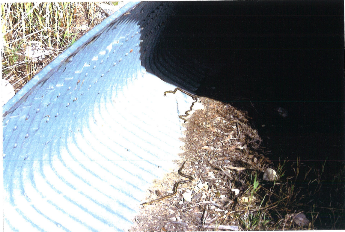
Plate 3: Snakes Travelling Along the Edges of the Culvert
