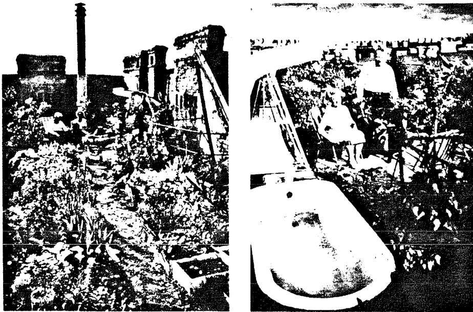
Figure 54: E.R. Finsches' Roof Garden, Vienna (From Lötsch, 1984.)
