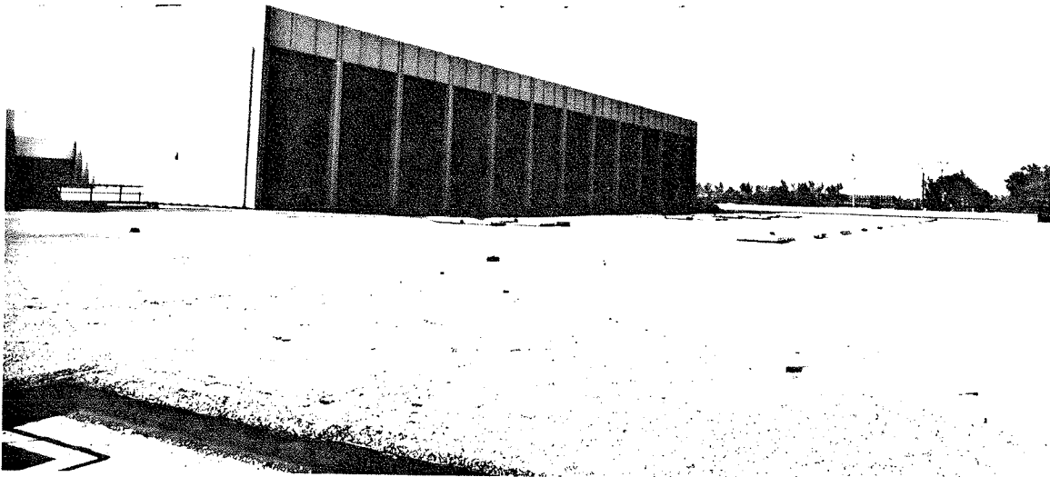
Figure 110: Frank Kennedy/Administration Studies Building Roof, University of Manitoba
