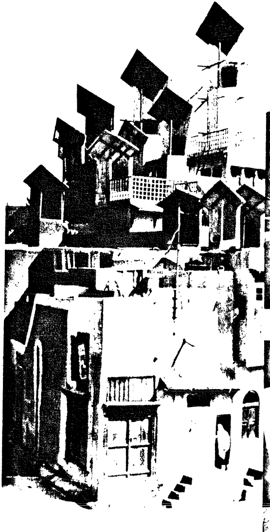
Figure 10: Roofs of Sind district of Pakistan (Note air scoops which channel breezes down into the homes. Photo from Rudofsky, 1964.)
