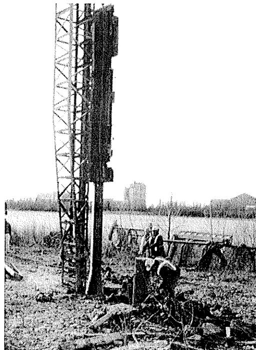
(b) Continued driving using a steel mandrel
