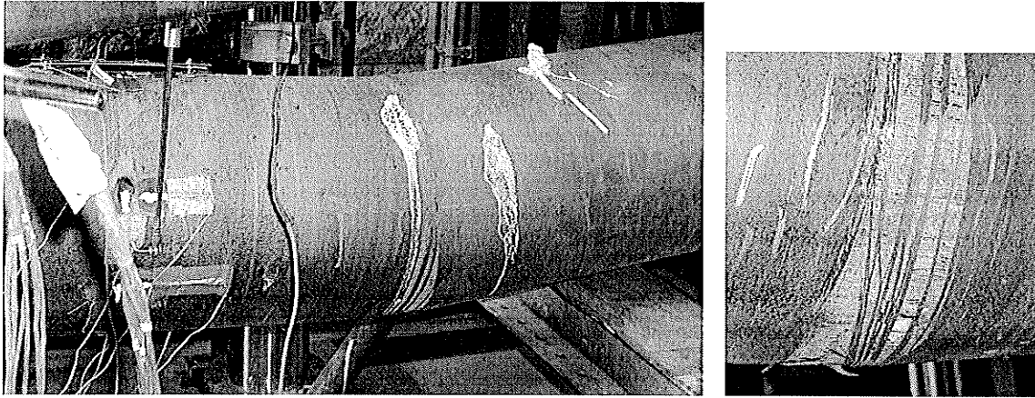
Figure 3-33 Failure mode of unspliced beams
