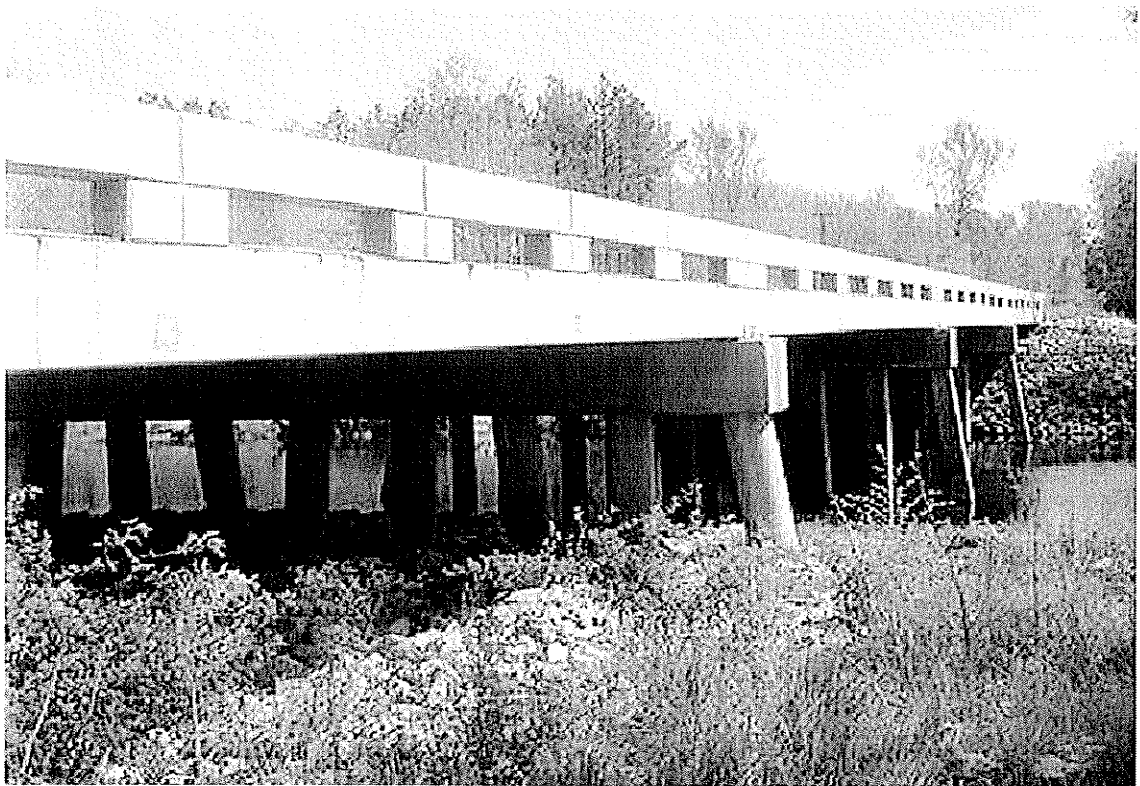
Figure 1-2 CFRTs in Route 40 Bridge pier, Virginia (Fam et al., 2003b)
