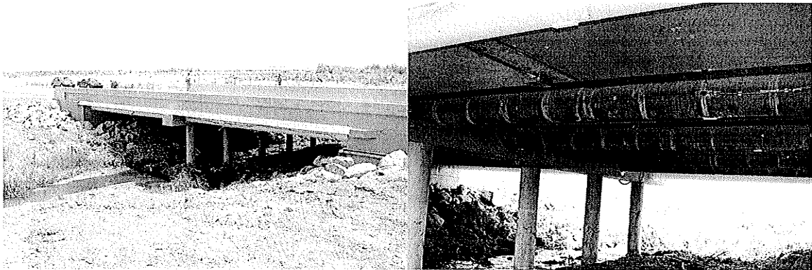
Figure 1-4 CFPT beams in Kings Stormwater Channel Bridge, San Diego, California (Seible et al. 1999)
