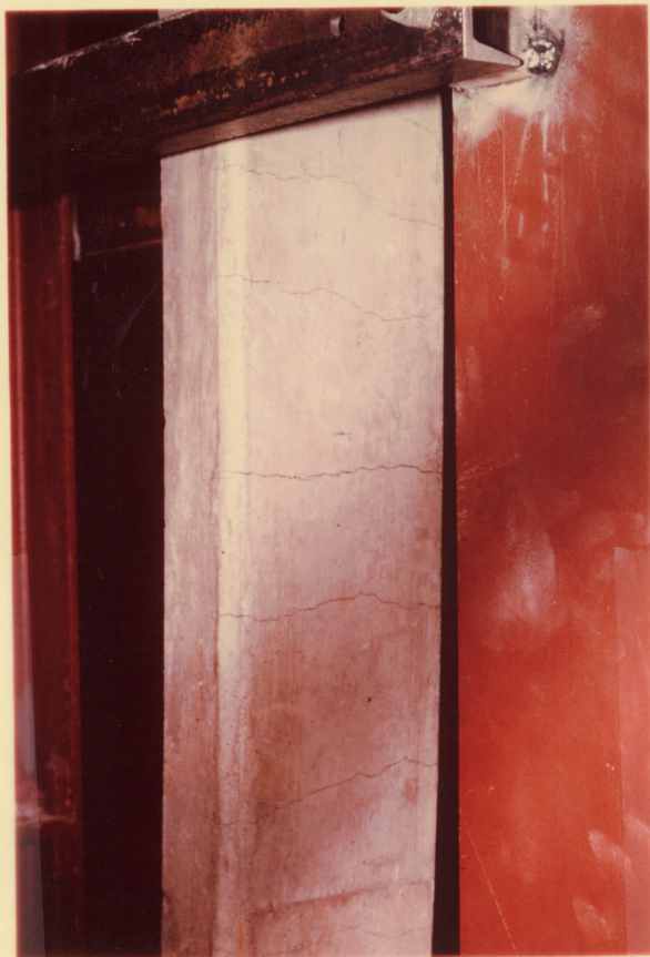
Column 2 B p Showing tensile cracks after buckling failure
