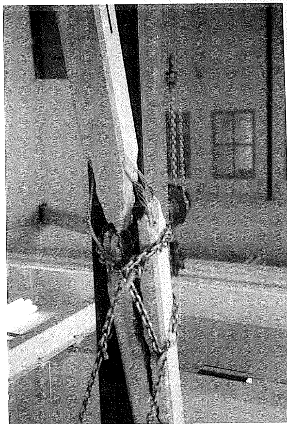
Column 2 B p Failure when supported at center
