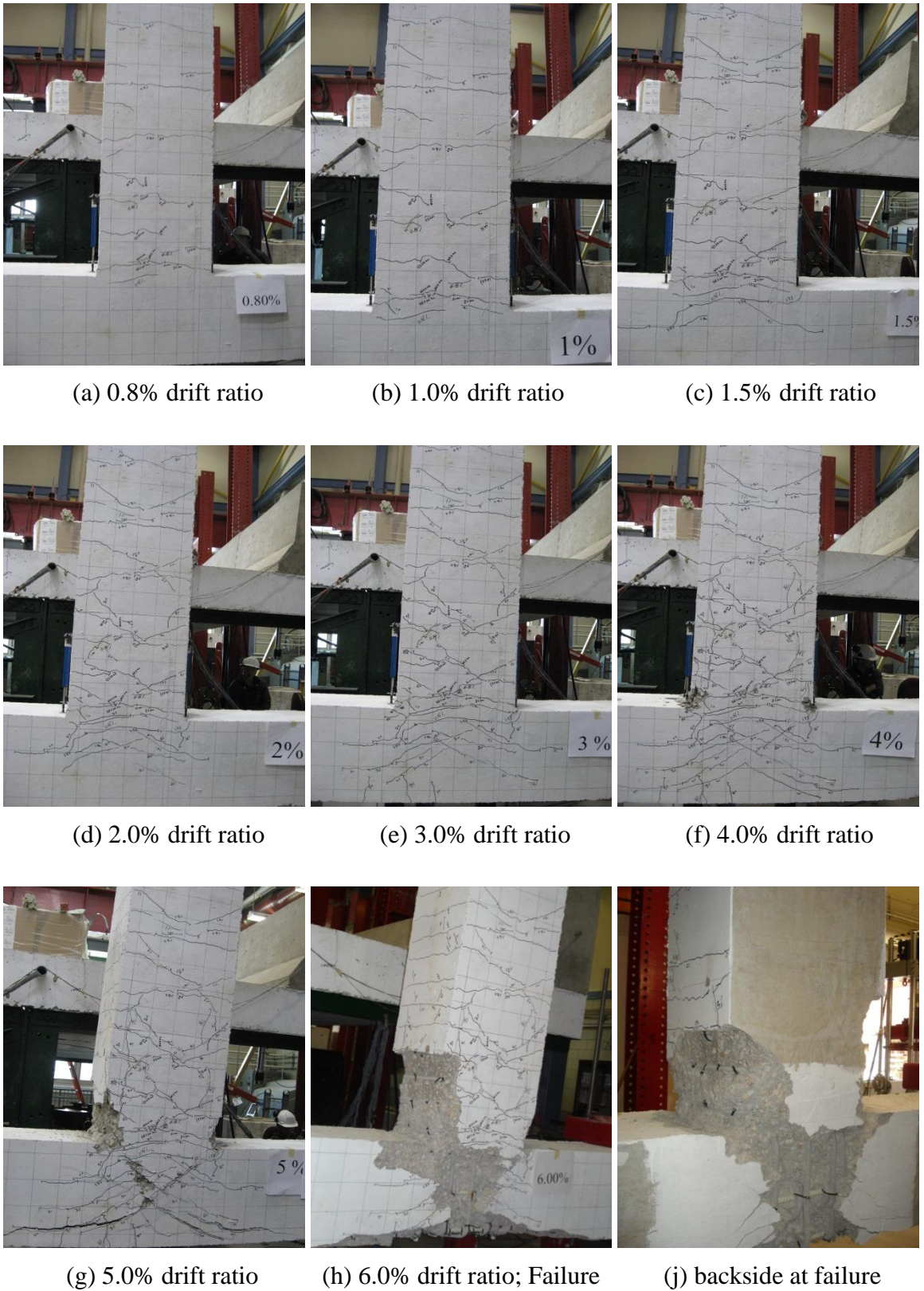
Figure 6.5: Cracking progression of Specimen II-30-0.85
