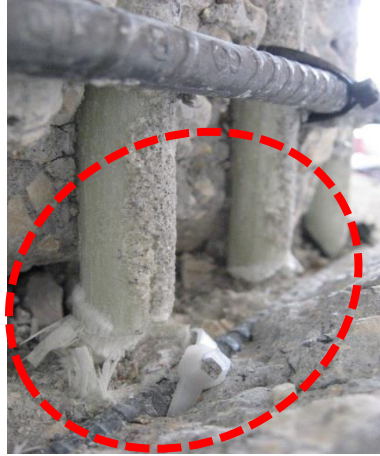
(k) Rupture of two bars and sand-coated surface shearing off
