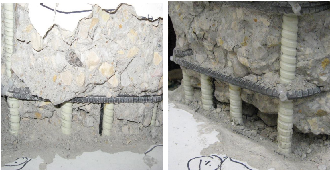
(b) Minimal damage for the deformed surface
