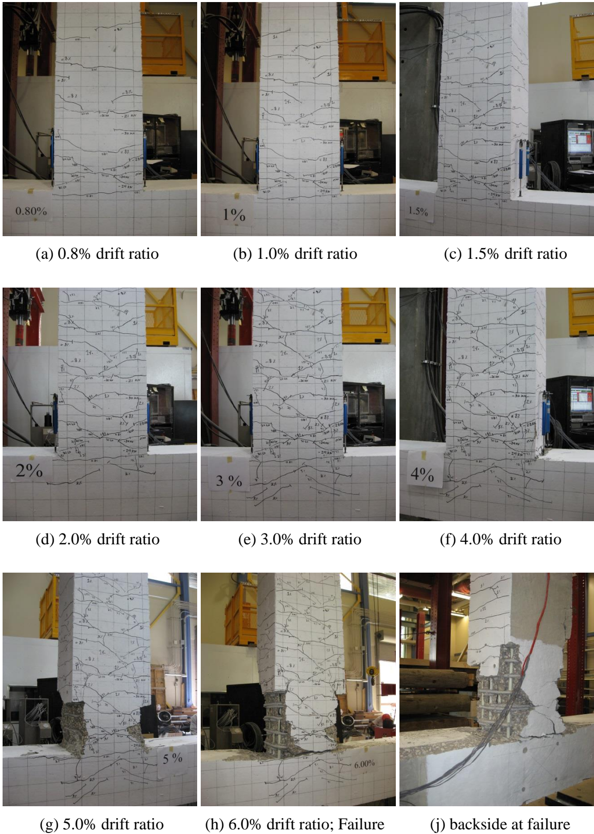
Figure 6.7: Cracking progression of Specimen II-60-0.70
