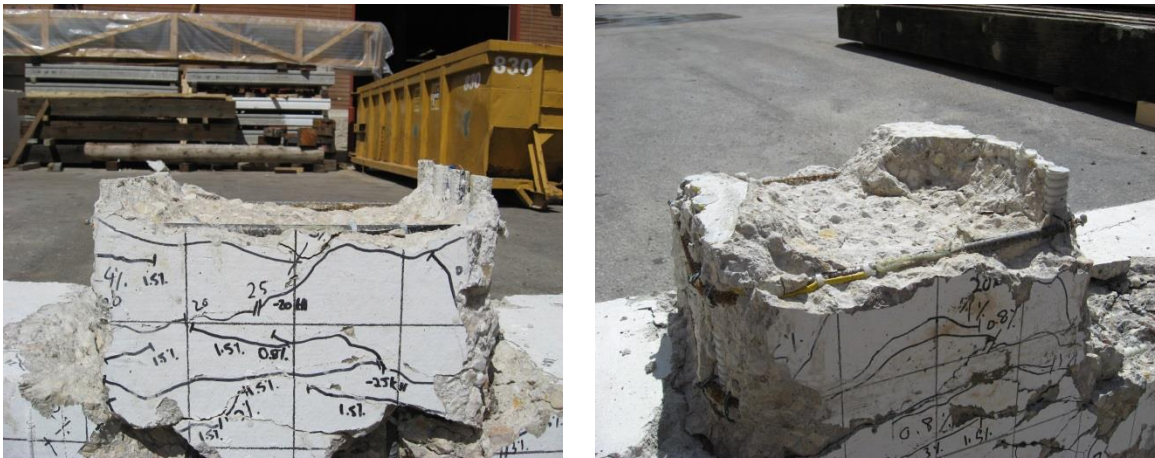
(a) Flat failure surface in beam section
