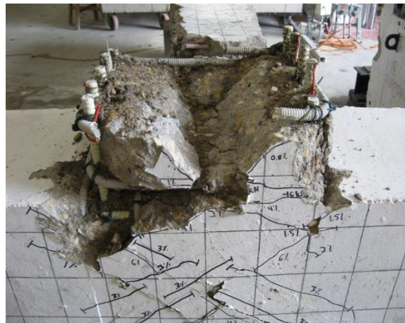
(b) Beam removed
