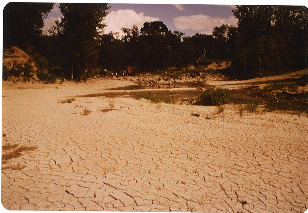
Plate 4 Dry Pool Upstream of Downstream Prototype Structure Looking Towards Crest - August 1981
