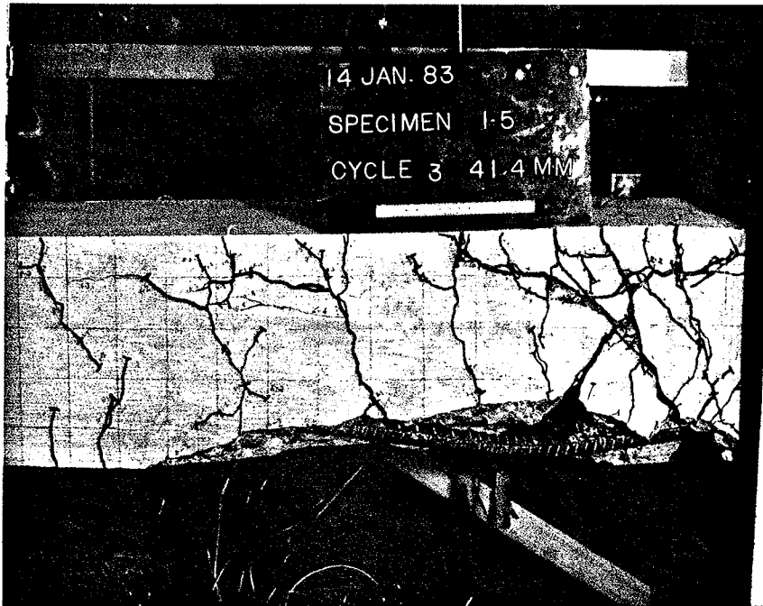
Fig. 4.21 CRACK PATTERN FOR SPECIMEN 1-5 AT 6\delta y/3
