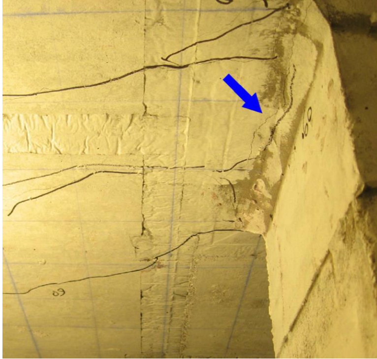
Figure 4.14: The formation of a crack at the inner column face in connection GRD-0.9-XX-0.4
