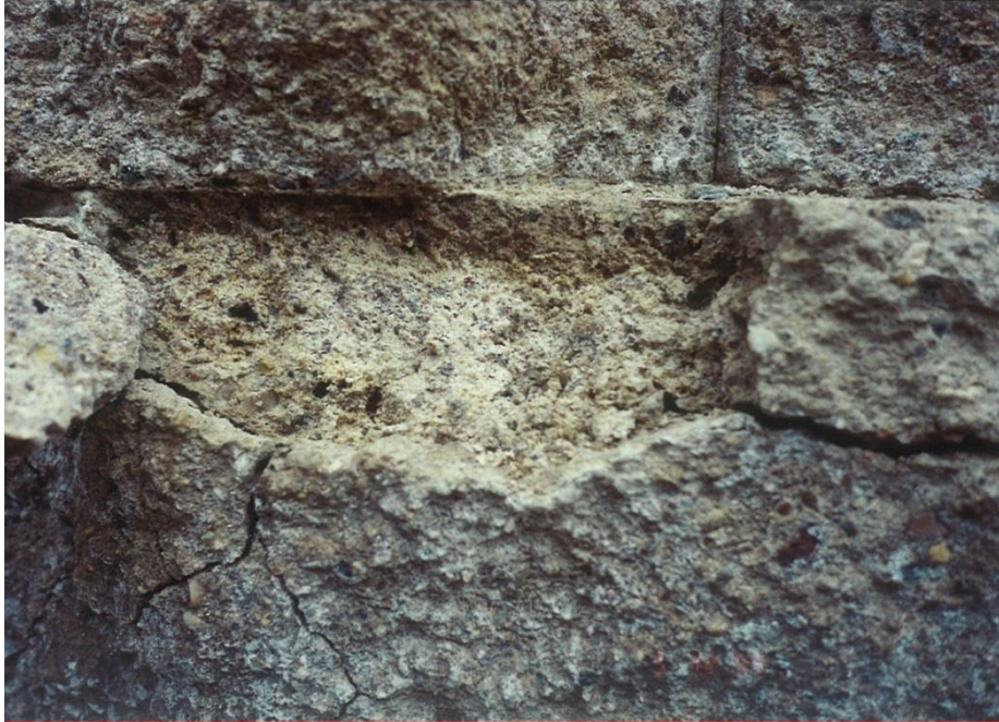
Figure 2.5: Visual features of precast concrete retaining wall units damaged by TSA (courtesy of Willems, T., CTLGroup, IL, USA).
