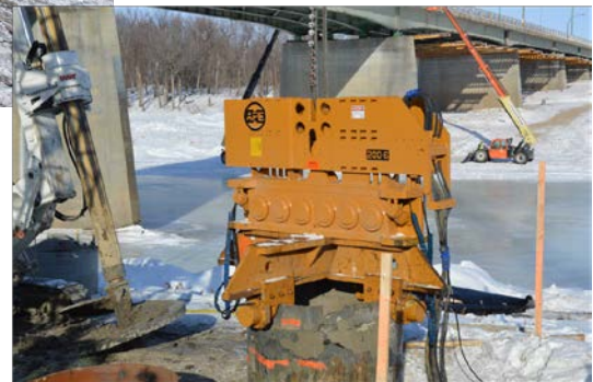
Figure 7-23 Installation of 25 m long rockfill columns on Red River. A vibratory unit (right hand photograph) was used to remove the casing and at the same time, compact a portion of the rockfill.
