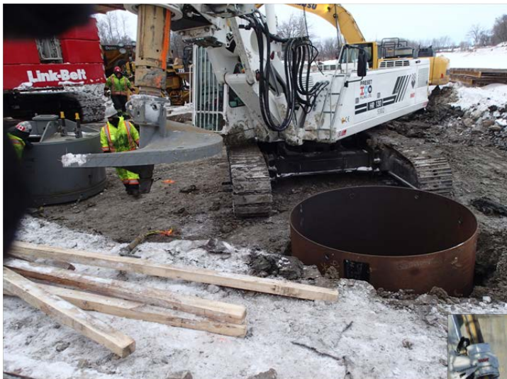
Figure 7-23 Installation of 25 m long rockfill columns on Red River. A vibratory unit (right hand photograph) was used to remove the casing and at the same time, compact a portion of the rockfill.
