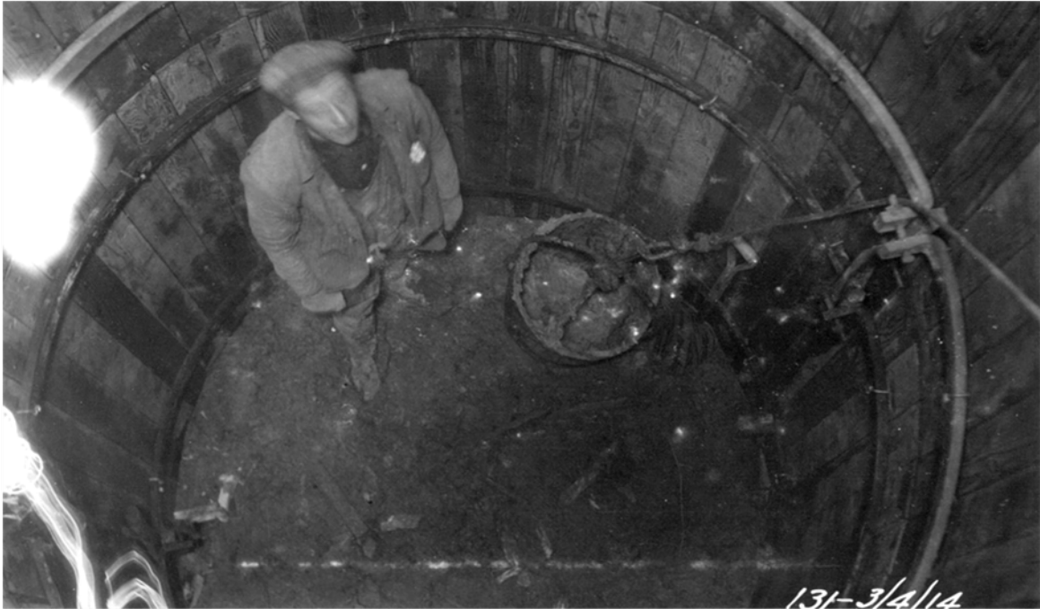
Figure 6-1 Sinking Chicago Well at the Transcona Grain Elevator (photo courtesy of B. Parrish Sr.)
