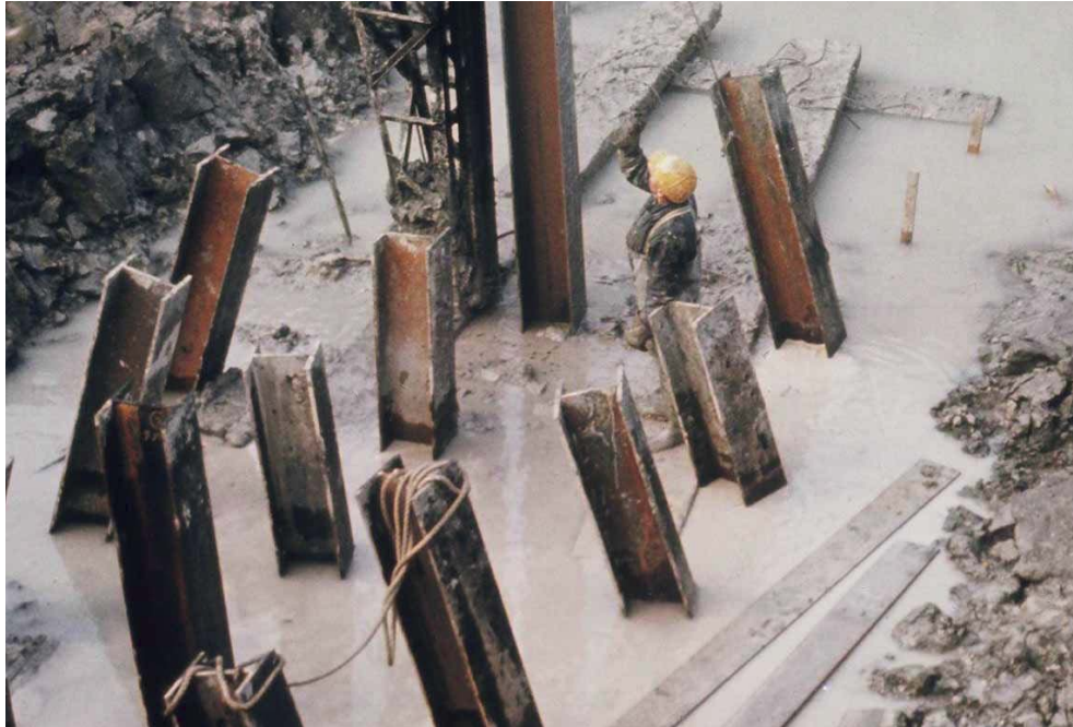
Figure 1-3 Pier foundations for CN Rail Bridge. Discharge into pier excavations for a rail bridge over the Red River Floodway reached 8,200 litres per minute accompanied by slumping of the excavation side slopes. Groundwater discharge was believed to be either from hydraulic fracturing of the clay or along the driven H Piles. Grouting was required to stop groundwater flow (from Render 1970).
