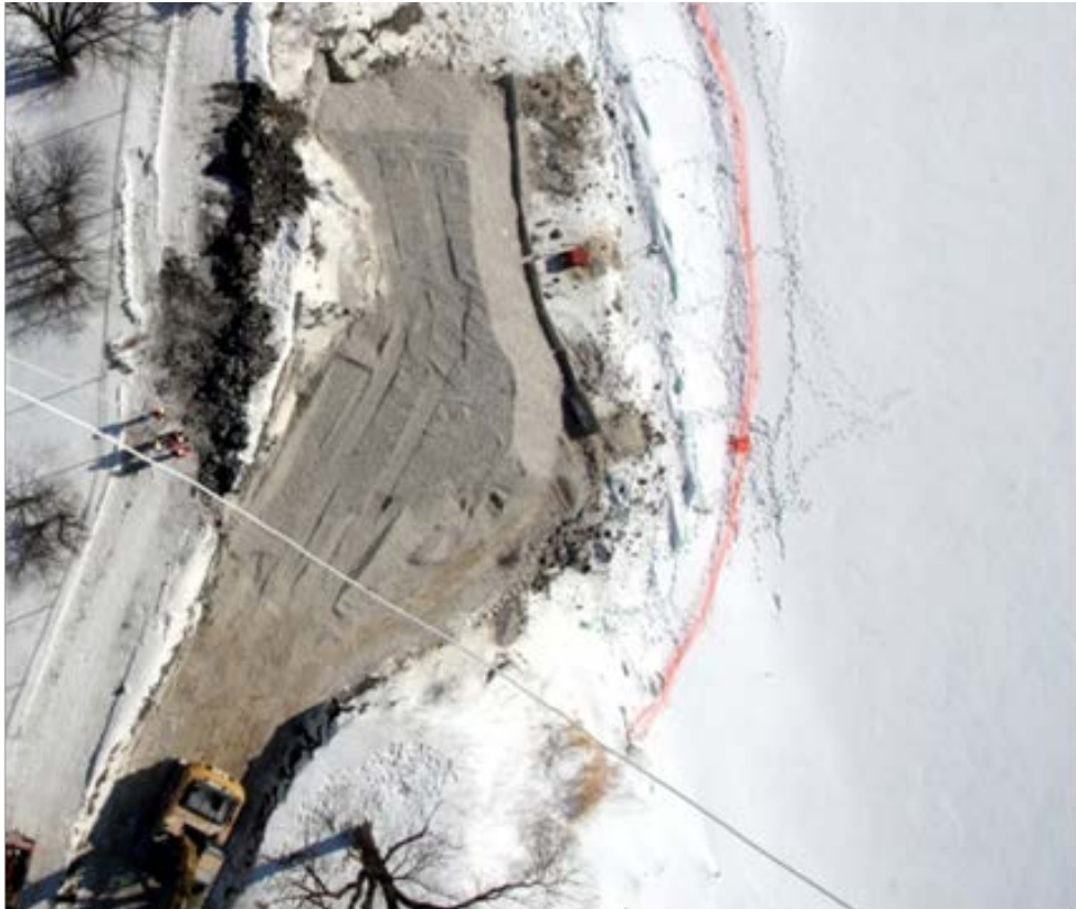
Figure 1-5 Aerial view of River Road test site. A full scale field test was carried out to determine the performance of rockfill columns for riverbank stabilization and optimize design parameters (from Thiessen 2010).
