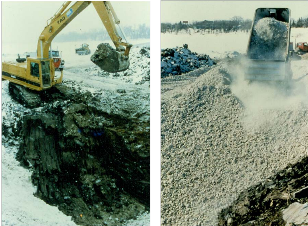
Figure 7-18 Shear key construction
