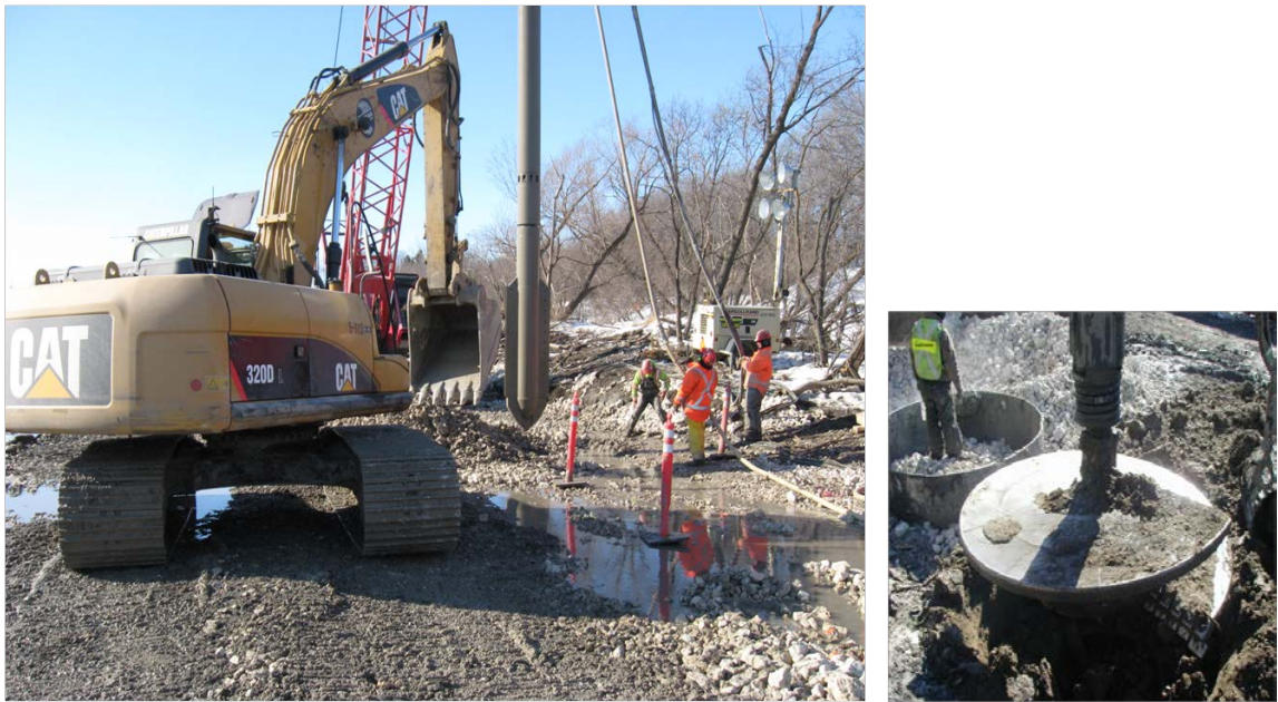
Figure 7-24 Drill rig auger (left photo) and compacting rockfill columns with Vibrolance
