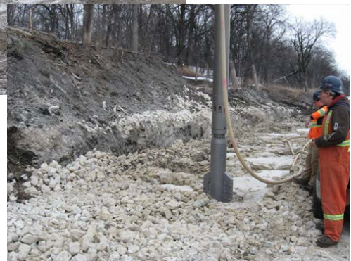
Figure 7-20 Compacting rockfill in shear key. Compaction is achieved using a vibratory probe mounted to an excavator on a grid pattern.
