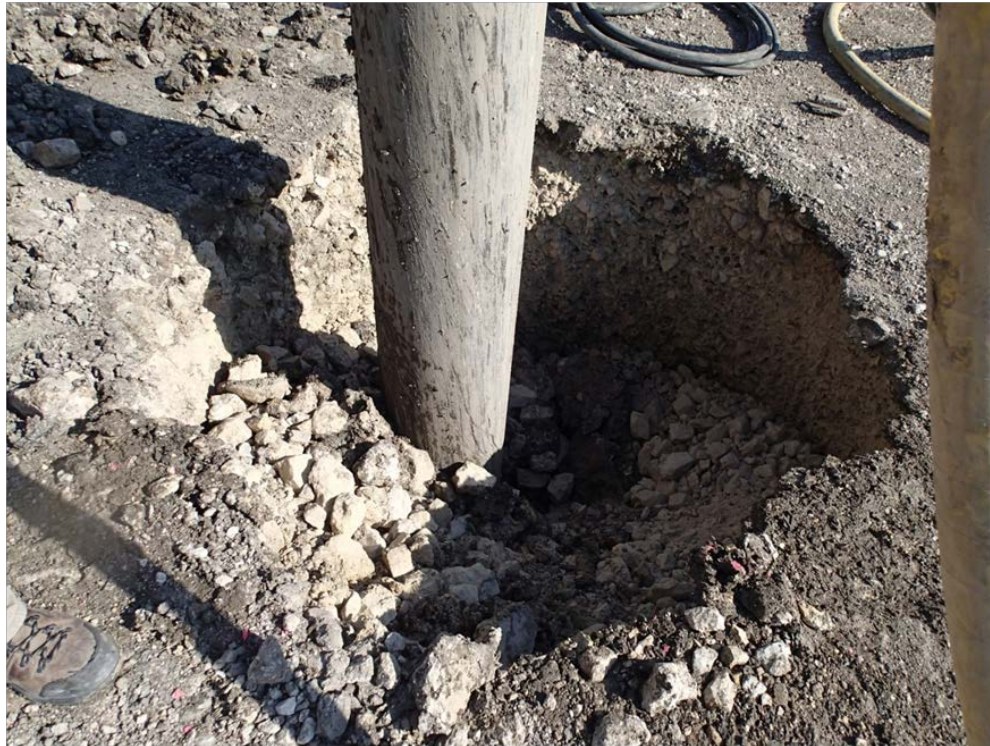
Figure 7-27 Rockfill dropping during compaction
