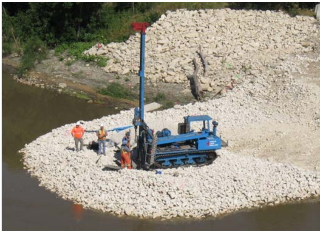
Figure 1-4 Auger drill rig operating off a gravel pad along the shoreline of the Red River in Winnipeg. Track mounted drill rigs can access sites that would otherwise be inaccessible to truck mounted drills.
