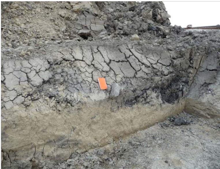
Figure 2-11 Basement excavation. The Upper Complex Zone often contains silt deposits of significant thickness and aerial extent. Here, the tan coloured silt layer can be seen across the side of a basement excavation in south Winnipeg. Also of note are large shrinkage cracks in the highly plastic clay after only a few days of exposure.
