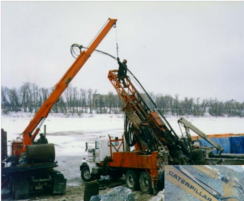
Figure 7-21 Installation of tie-back anchors in shear key
