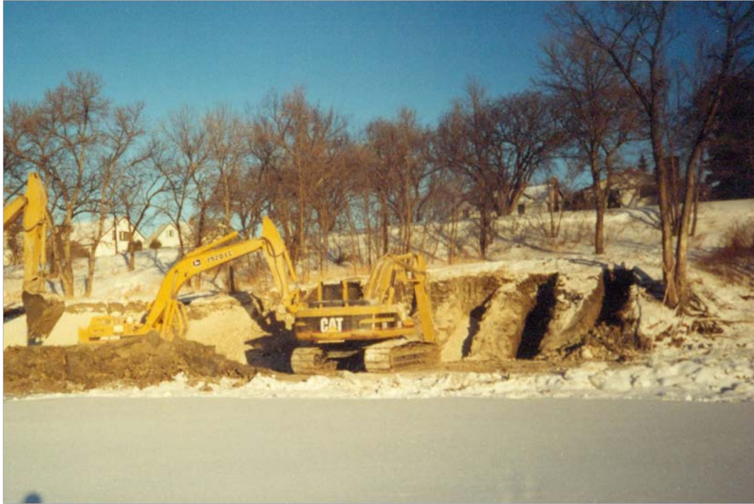
Figure 7-19 Construction of granular ribs
