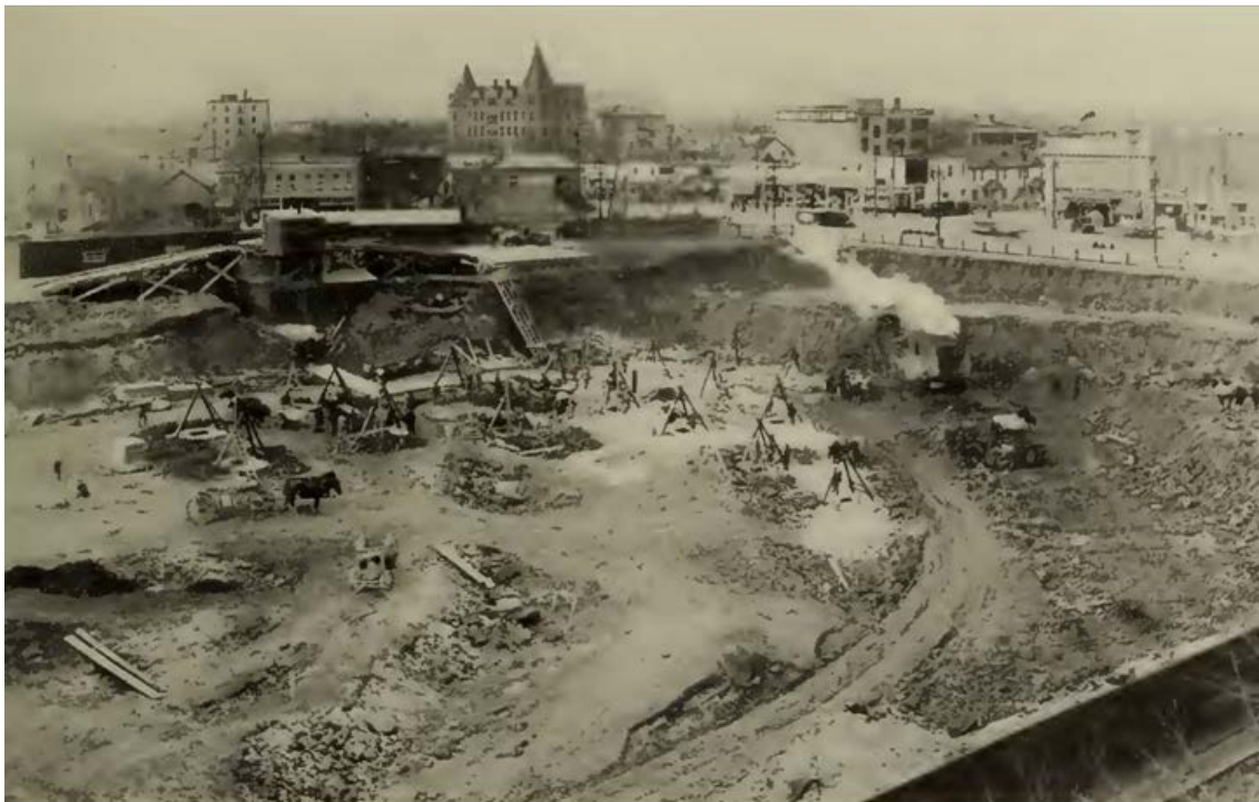
Figure 6-2 Excavation for the Hudson's Bay Store in Winnipeg (c. 1926) A total of 151 caissons were advanced to the limestone bedrock and no building at the time had had a higher percentage of bad caissons (Fosness 1926)
