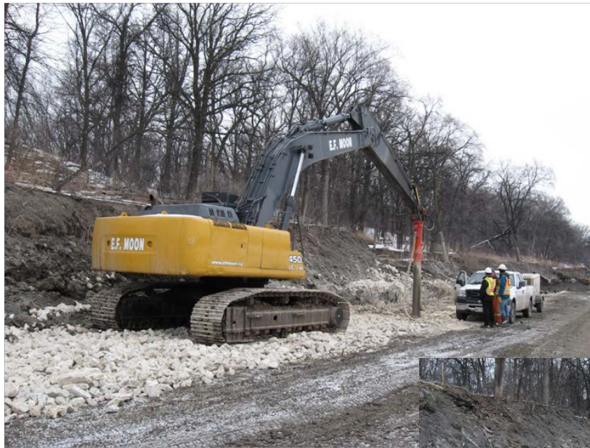
Figure 7-20 Compacting rockfill in shear key. Compaction is achieved using a vibratory probe mounted to an excavator on a grid pattern.
