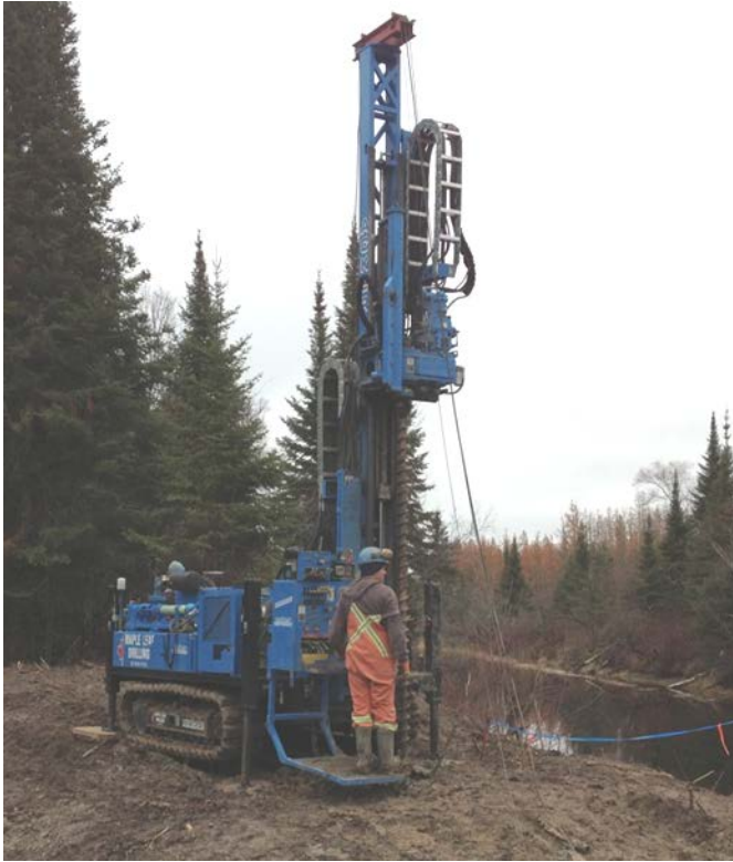
Figure 4-3 Track mounted drill rig with 125 mm diameter solid stem augers. Depending on the height of the mast, up to 3 metres of auger can be pulled straight out of the borehole for sampling purposes.
