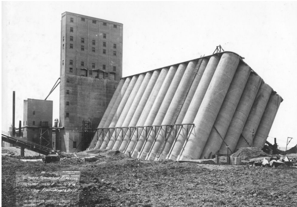
Figure 1-1 Elevator binhouse after failure (c.1914). The foundation failure and righting of the Transcona Grain Elevator is recognized as a truly remarkable case history made famous by its collapse after bearing pressures exceeded the limiting shear resistance of the clay foundation. The structure was successfully righted and remains in service today (photo courtesy of Bill Parrish Sr.).
