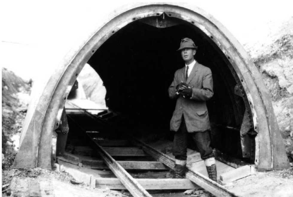
Figure 1-2 Construction of the Shoal Lake Aqueduct (c.1916). Designers were faced with nearly unimaginable variability in ground conditions along nearly 100 miles from Shoal Lake to Winnipeg through the harsh geological environment left by the remnants of glacial Lake Agassiz (photo courtesy of the City of Winnipeg).
