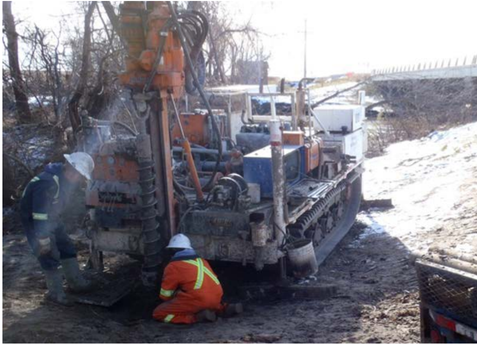
Figure 4-5 Track mounted drill rig equipped with hollow stem augers.
