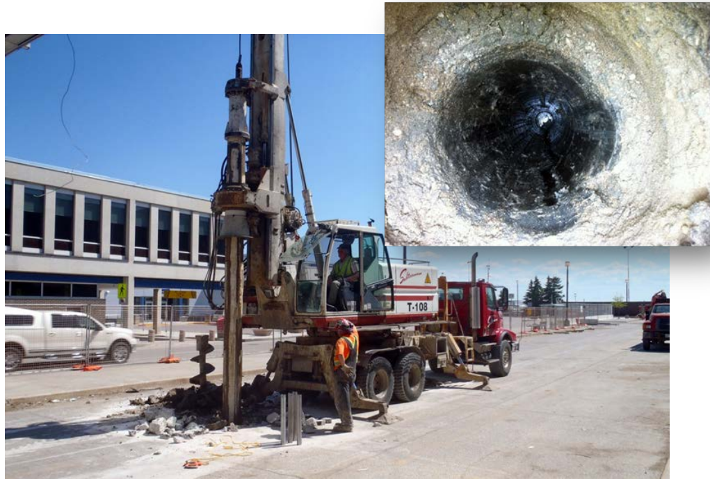
Figure 4-4 Piling Rig Borehole. The auger has been removed and a Shelby tube is being pushed. The photo inset illustrates the ability to visually assess soil and groundwater conditions in the open hole. Surficial gravel fill is visible near surface and water can be seen reflecting light at the bottom of the hole.
