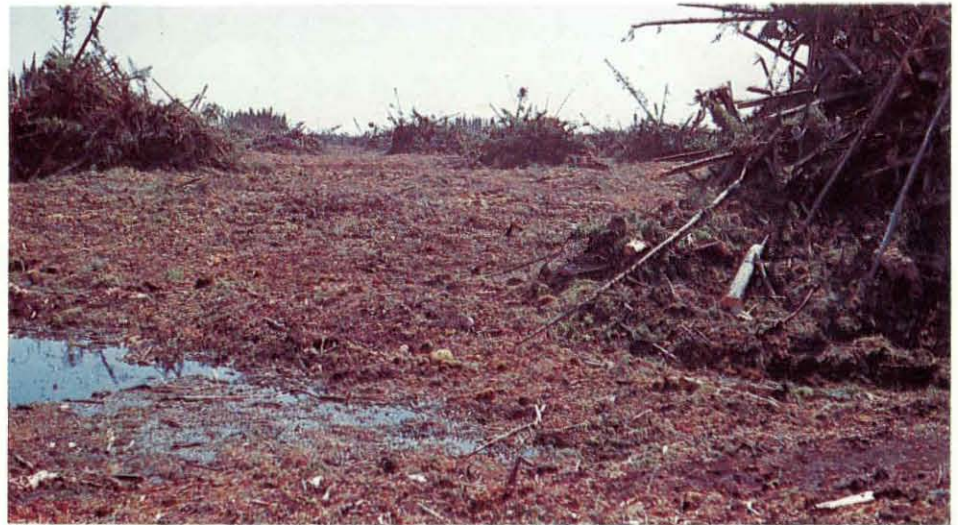
Clearing Piles, Jenpeg (R. J. Lay).
