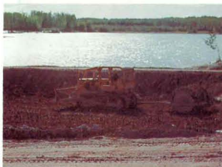
Kiskitto Dam, Construction (R. J. Lay).
