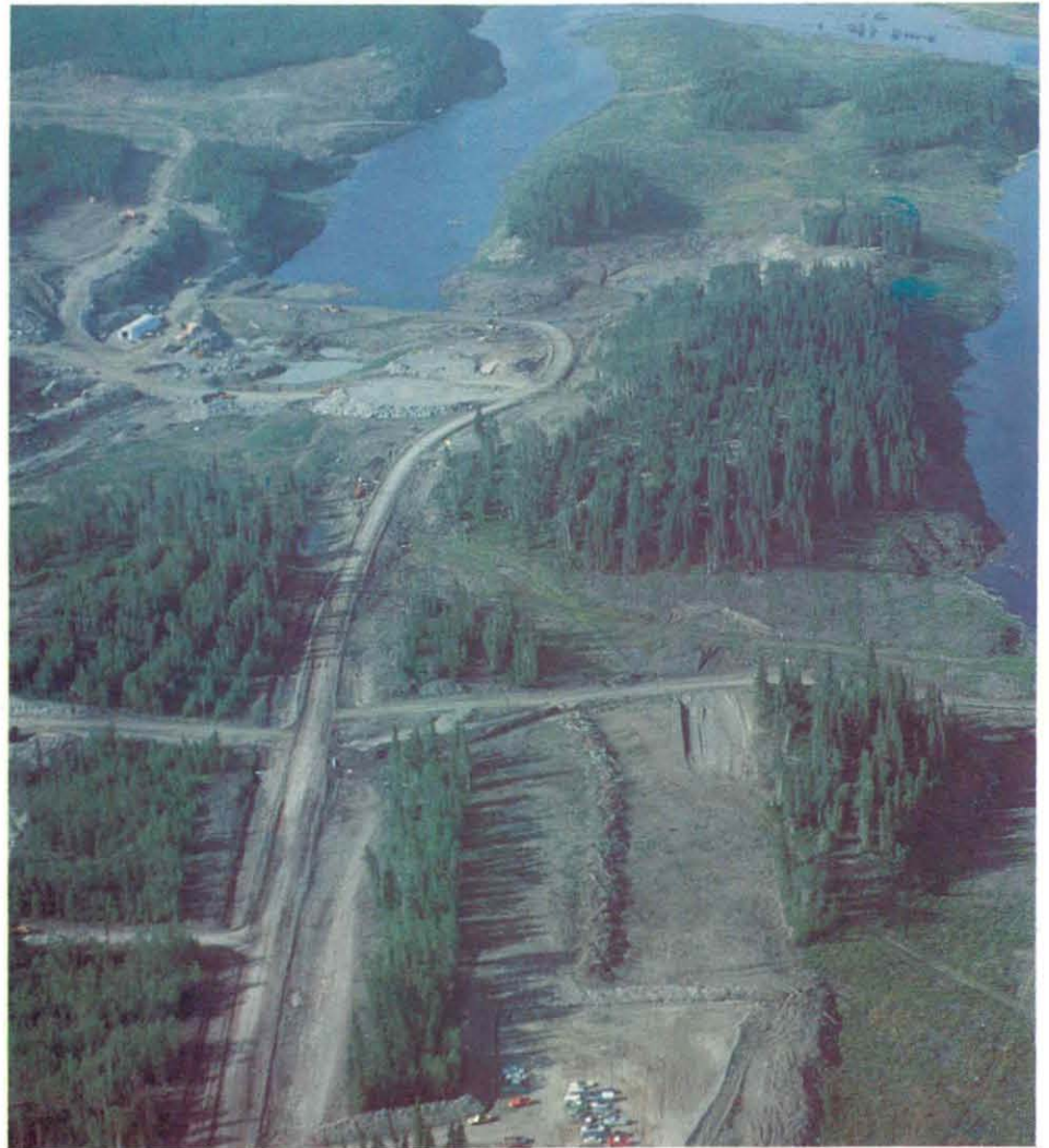
Construction Activity at Notigi (Study Board).
