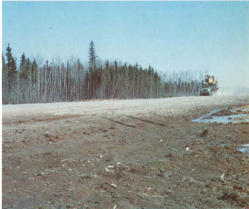
Jenpeg Access Road (R. J. Lay).
