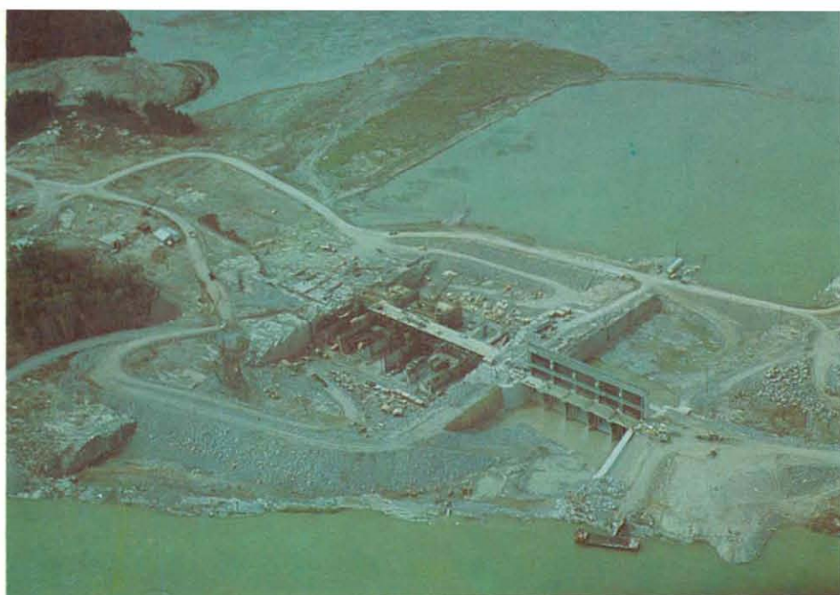
Jenpeg Construction, Summer 1974 (Study Board).
