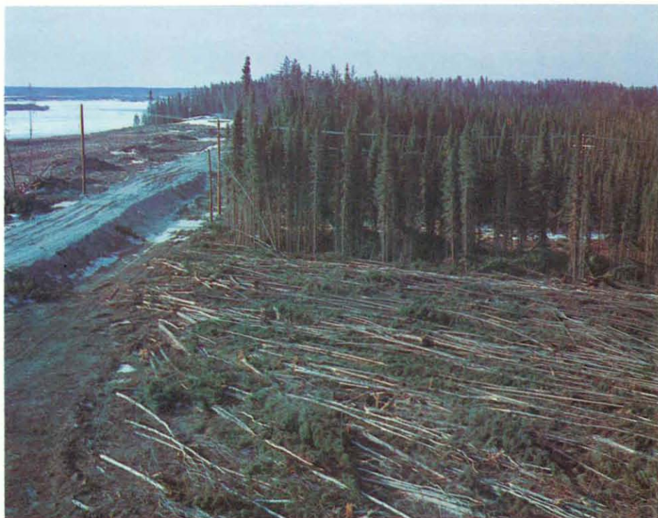
Timber Clearing near Jenpeg (R. J. Lay).
