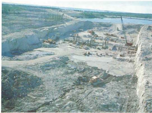
Construction at Missi Falls, Summer 1974 (Manitoba Hydro).
