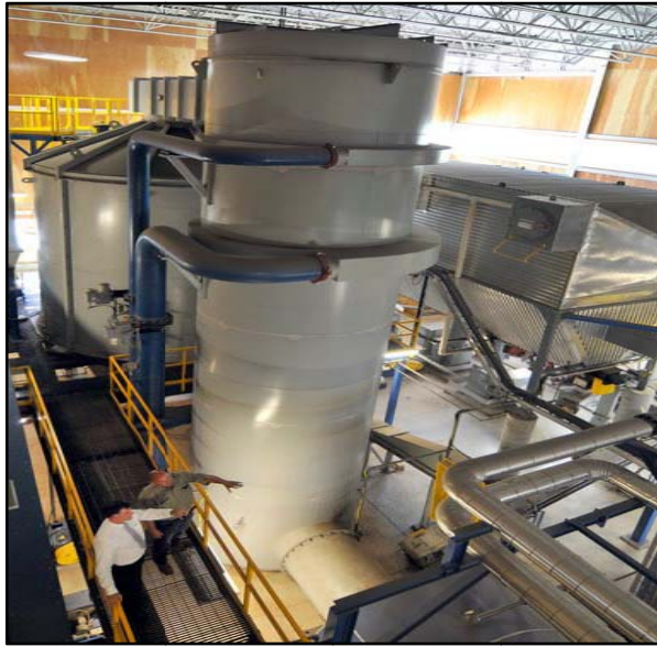
Photo 5-1: Wood biomass heating plant (2 MW) in University of Northern BC, Prince George (Source: Nexterra, British Columbia).
