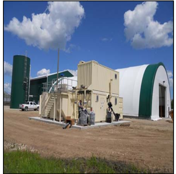
Photo 5-2: BioMax 100 micro-gasification CHP system in the Pineland Forest Nursery, Manitoba (Source: NRCan, 2014).
