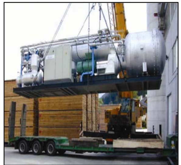
Photo 5-4: A biomass-fired ORC unit (Source: Dong et al., 2009).
